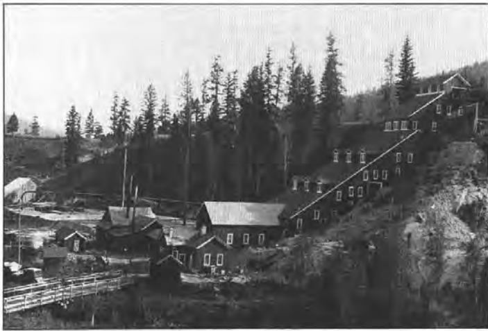
Patsy Clark mill at the Republic mine, 1898.
