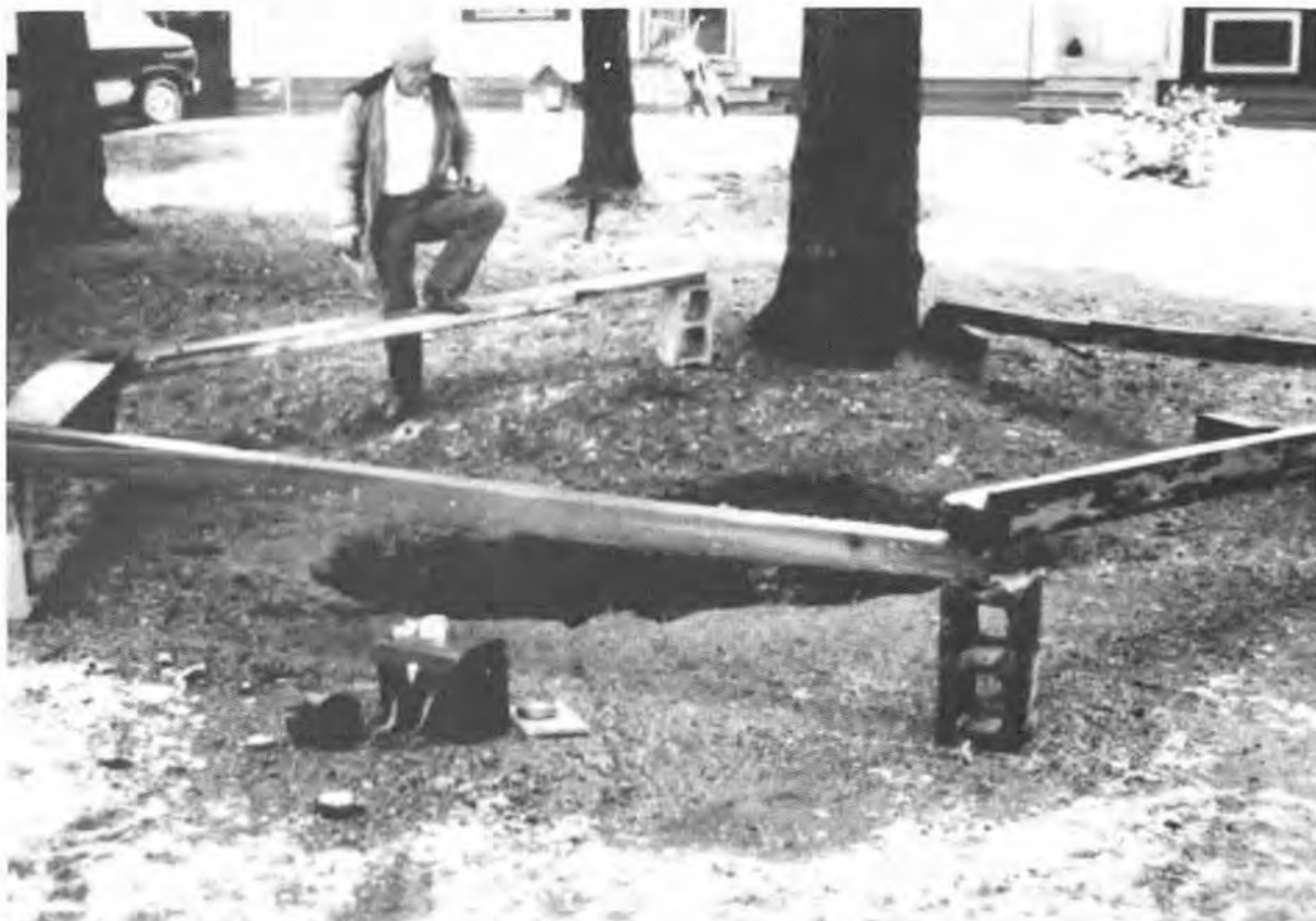
This cave-in occurred in 1979 over shallow mine workings at the Wonder mine near Ravensdale. (See article, p. 3.)
