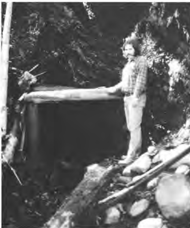
Figure 2. Original adit, Discovery seam, Glacier coal field. (Photo by Ellis Vonheeder, DNR)
