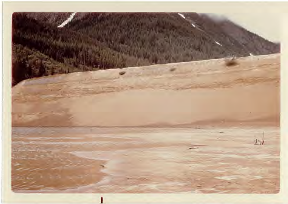
Photo No. 2. — East face of tailings pile number 2 viewed from surface of pile number 3. Bank is about 75 feet high. Note wind deposited material at angle of repose on this lee slope. Note also the willows and unidentified brush rooted in talus material used as diking near upper level of the dike. Thimble berry and a few conifers are present at this same level on the other side of the pile.
