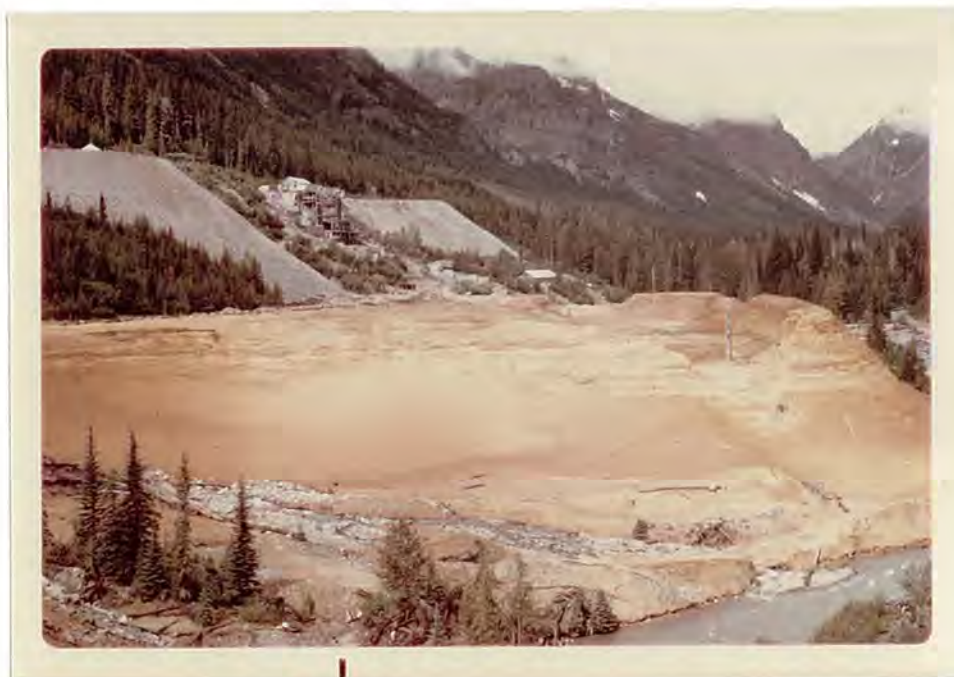
Photo No. 1. — Mill tailings pile number 1 with mine dumps in background, looking west, up valley of Railroad Creek. This pile was partially hydrauliced (1947), remilled, and pumped underground as sand fill. This operation was apparently responsible for presence of tailings in the creek bank as no such condition exists along the other tailings piles.
