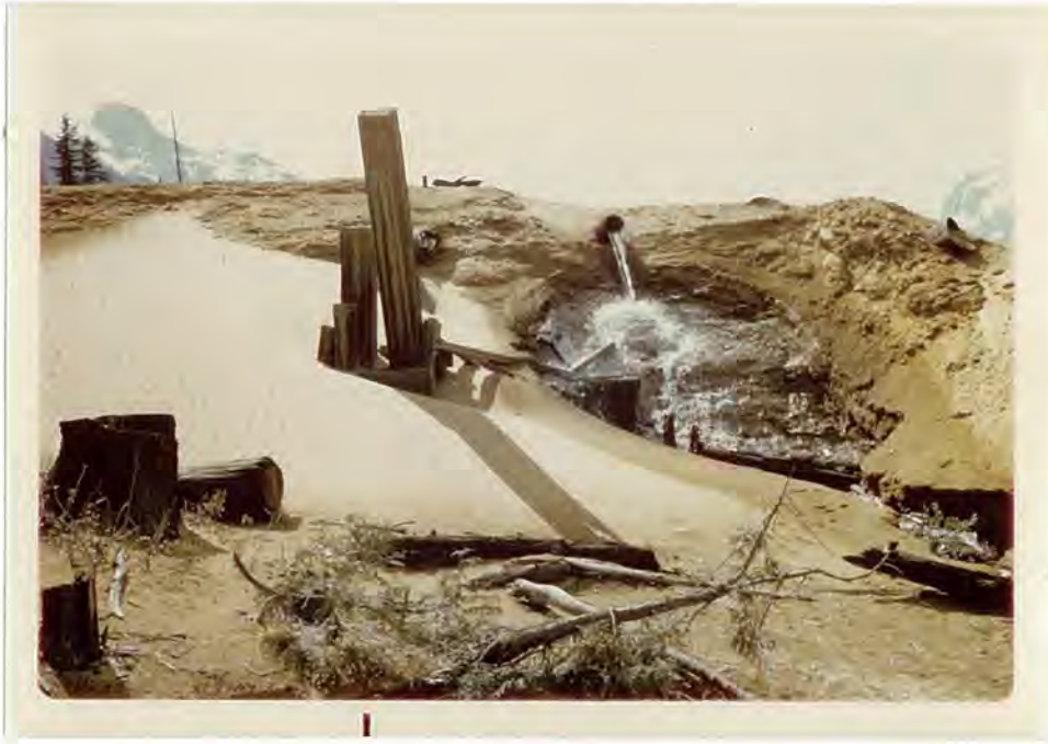
Photo No. 4. — East edge of tailings pile number 1 (photo is "off-color"). This picture shows the relative resistance to erosion of undisturbed oxidized tailings compared to wind deposited tailings. Culvert discharging stream of about 3 square inches in cross section falling 4 feet onto sloping surface of stratified tailings. Note the relatively minor erosion considering that this stream has apparently flowed, at least intermittently, for at least 20 years. No turbidity noticeable in the runoff.
