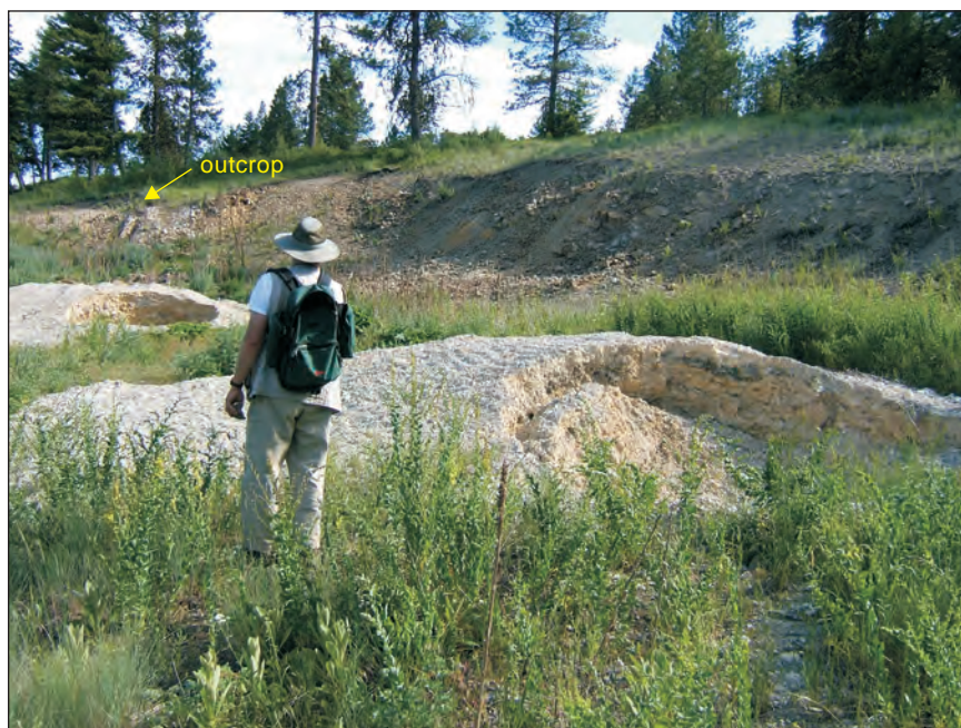
Figure 11. Subsidence over backfilled stope openings at the Ben Hur mine. Vein outcrop at upper left. View is along strike to the southeast.
