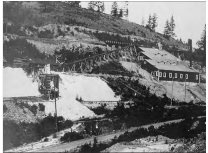
Figure F3. Overview of the San Poil mill and mine site circa-1916. The main haulage tunnel is located at the center left at the terminus of the surface tram running upslope to the crusher building. Note the rock dump overflowing the rail tracks next to the loading bin, left center. Ben Hur mine is off photo at right. Eureka Creek and Knob Hill mine road is at the bottom. View is to the west. Photo courtesy of Ferry County Historical Society.
