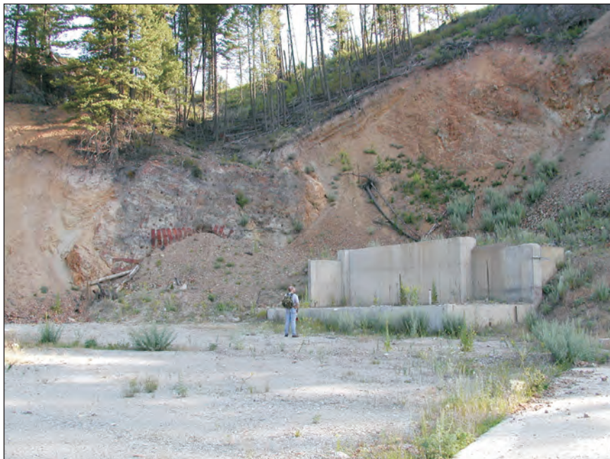
Figure 13. Plugged and abandoned Golden Promise ramp site, 2001. The portal is to the left of the geologist, near the foundation of a former dry house and storage building.
