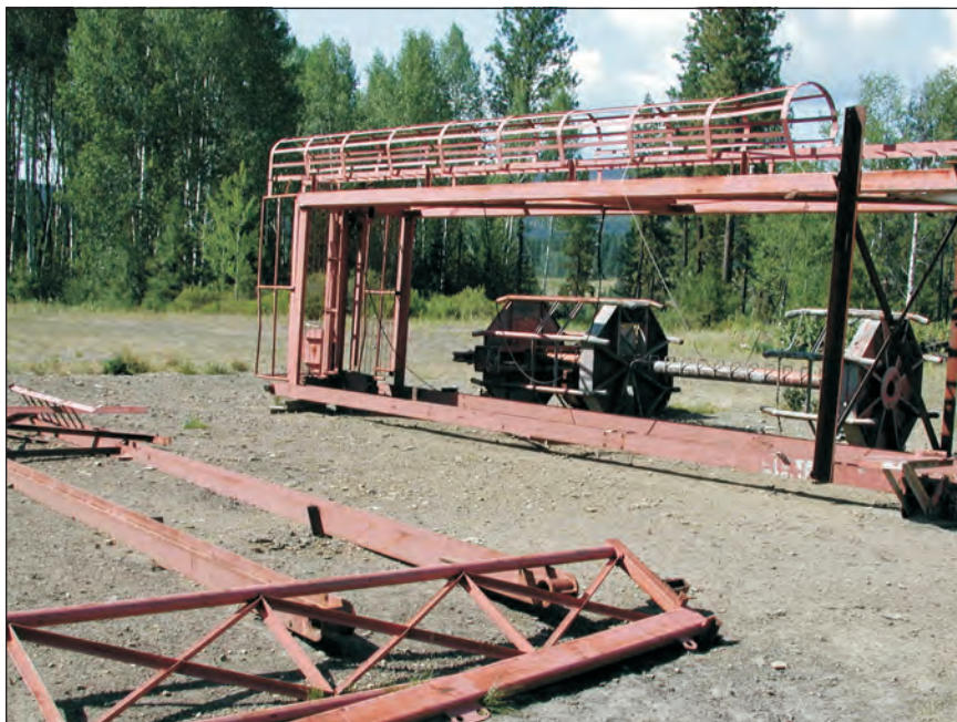
Figure 19. Men and materials cage and equipment used in the Golden Promise vertical shaft, 1986–1995.
