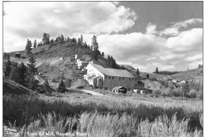
Figure F4. Knob Hill mill circa-1949. Original mine adits are located on the hillside above and to the left of the mill. The Knob Hill mine No. 2 inclined shaft is located over the ridge at the far left. View is to the north. Photo courtesy of Ferry County Historical Society.
