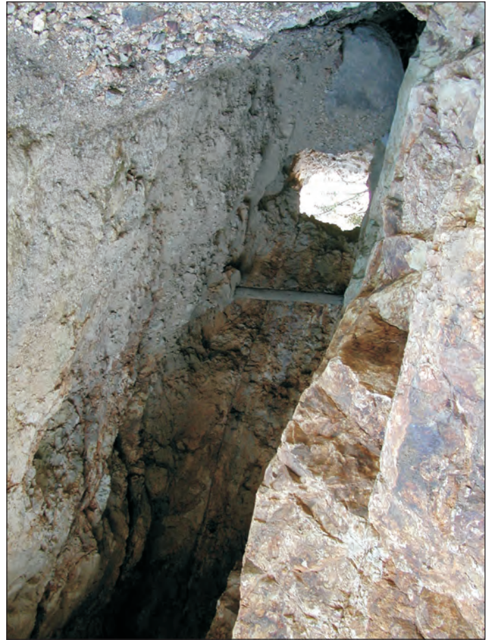
Figure 6. Stope opening at the surface at the Quilp mine. Eight-foot timber at center for scale.
