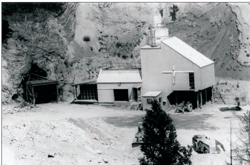
Figure 12. Golden Promise ramp portal, 1995. View is to the east.
