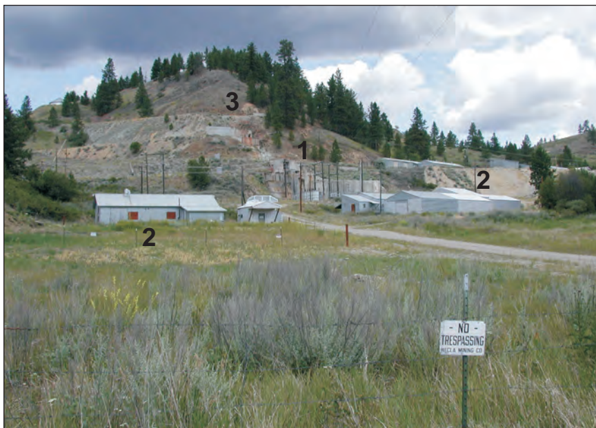
Figure 18. Hecla's Knob Hill mine site 2001, showing mill foundations (1), shop buildings (2), circa-1920 adits on Knob Hill (3). View is to the north.
