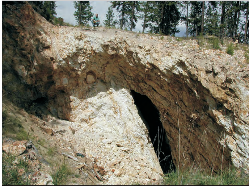
Figure 4. Vein outcrop and open stope at the Republic mine. Geologist at top left center for scale. View is to the northeast.
