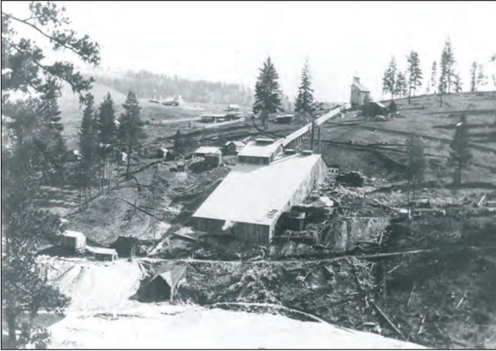
Figure F5. Overview of the Mountain Lion mill and mine site circa 1900. A covered tramway runs from the vertical shaft head frame (top right) to the mill. The 1260-foot southeast-bearing adit is located adjacent to the dry house and compressor buildings at the far left bottom. Note the mill tailings spreading out on the flood plain of Swamp Creek, which flows from left to right. View is to the east. Photo courtesy of Ferry County Historical Society.
