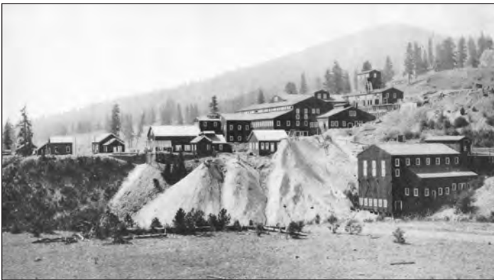
Figure F2. Republic Consolidated Mining Company's 'Red' mill at the Republic mine, probably circa 1915–1920 after the property was in receivership. The boiler smokestacks and the surface tramway that carried ore from the sampling mill at the lower right to the crusher building at top right have been torn down. Patsy Clark mill ruins are out of the photo to the left. The various stacks of white material in the center of the photo are waste rock and mill tailings deposited on the west bank of Granite Creek, which flows from right to left. The brush and road in the foreground lie on the east bank. The discovery site of the Republic vein and prospect trenches are out of the photo at the top right. View is to the southwest. Photo courtesy of Ferry County Historical Society.
