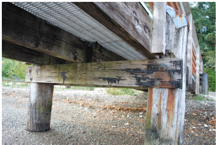
Above: Example of creosote-treated pilings and framing in a dock. Photo: Lalena Amiotte/DNR.
