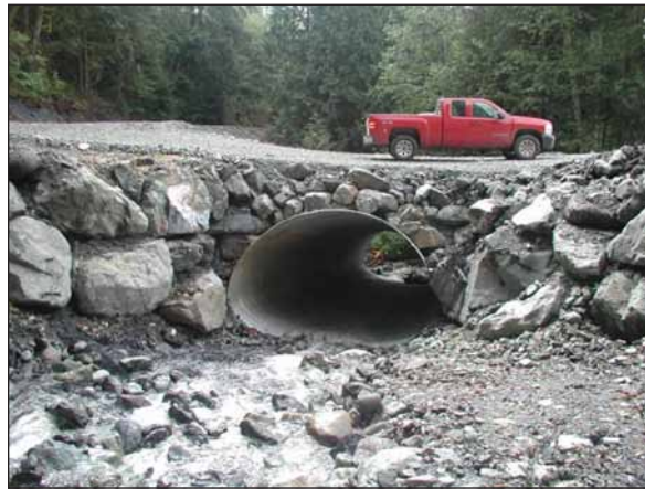
Figure 4.10. Dipped rock fills result in stable road prisms at stream crossings. Note the large-arch culvert, heavy-rock armoring, and minimal fill over the culvert.
