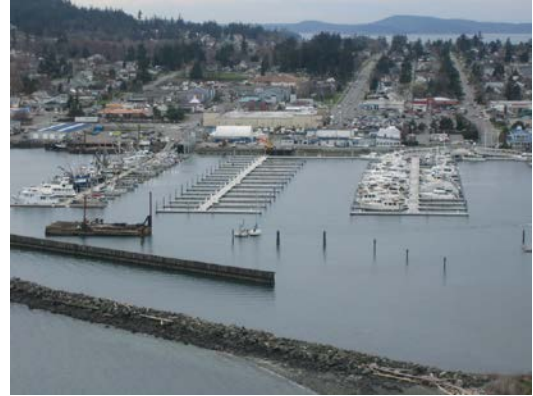
Rubblemound breakwater structure horizontal to marina facility Photo: DNR staff.
