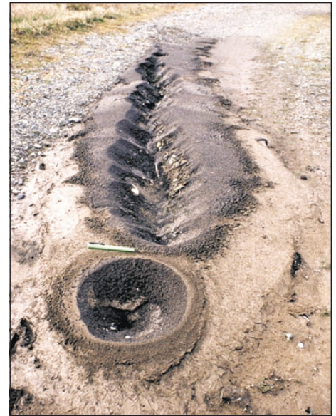
Figure 20. View of sand blows from an east-west trending crack at the Nisqually National Wildlife Refuge (Nisqually River delta). The crack is located on Center Road about 220 yards northwest of the twin barns. The ejected sediments contain abundant crystals, as well as lithics and pumice, of Mount Rainier andesite. Marker pen is for scale (5.3 inches). Photo by Pat Pringle, March 4, 2001.
