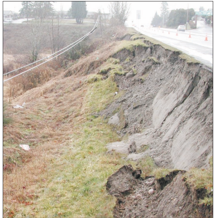
Figure 9. Landslide on Martin Way between Ensign Road and Pattison Street in Olympia. View to the east. The slide took out some utility poles but the wires remained intact. Photo by Karl Wegmann.
