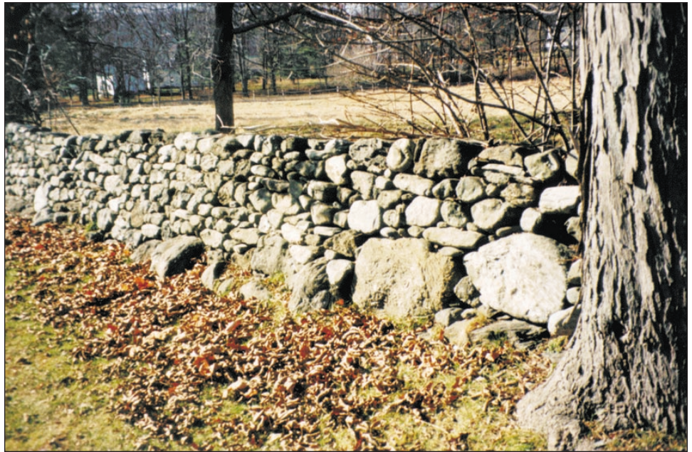
Figure 2. A dry-stacked stone wall in Connecticut. Notice the rounded edges of the stones, the wide base, and the placement of the largest stones at the bottom of the wall. Photo by Eric Gerstel.
