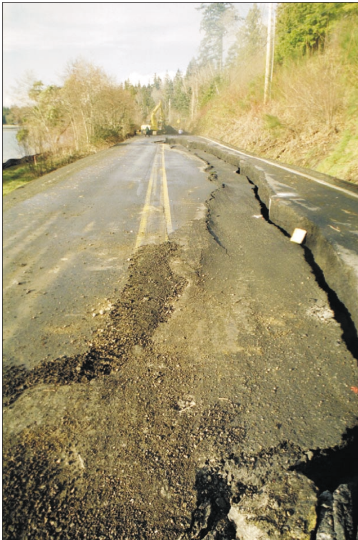
Figure 9. Landslide on Martin Way between Ensign Road and Pattison Street in Olympia. View to the east. The slide took out some utility poles but the wires remained intact. Photo by Karl Wegmann.
