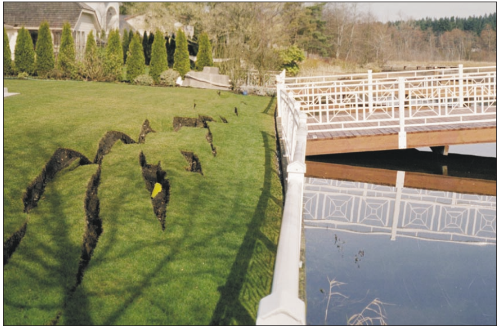
Figure 7. View of a lateral spread in a residential yard on Long Lake east of Lacey. The fence is attached to a retaining wall at the edge of Long Lake. This lateral spread occurred in a manmade fill that is superimposed on peat and lacustrine sediments. The failure pattern is controlled by lower root-strength between strips of new sod and by the retaining wall, which was down-dropped and back-rotated. Photo by Bill Lingley.
