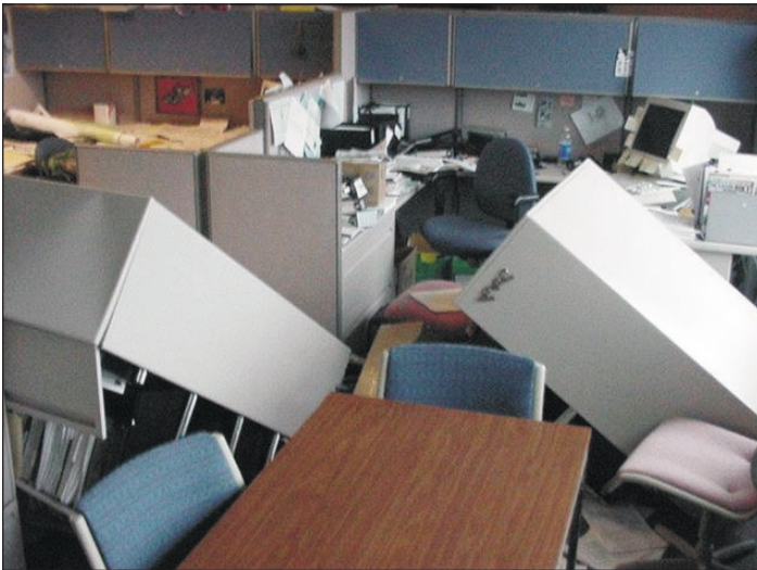
Figure 3. Sixth floor cubicle damage. Photo by Ray Lasmanis.
