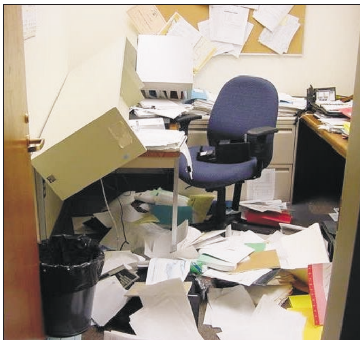
Figure 1. Sixth floor cubicle damage. Photo by Dennis Heryford, Department of Natural Resources.
