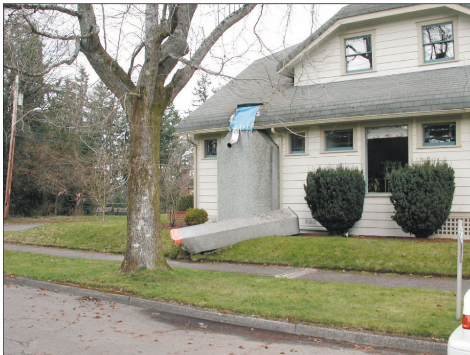
Figure 13. Chimney topple at a private residence in the South Capitol area, Olympia. Photo by Karl Wegmann.
