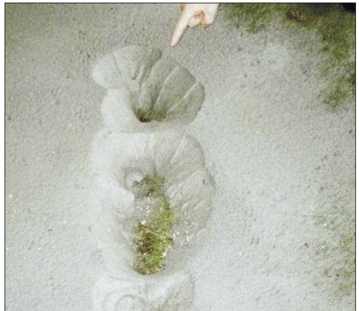
Figure 2. Sand boils (incipient lateral spread) at the Port of Olympia in an area with several boils and extensive cracking. Photo by Hank Schasse.
