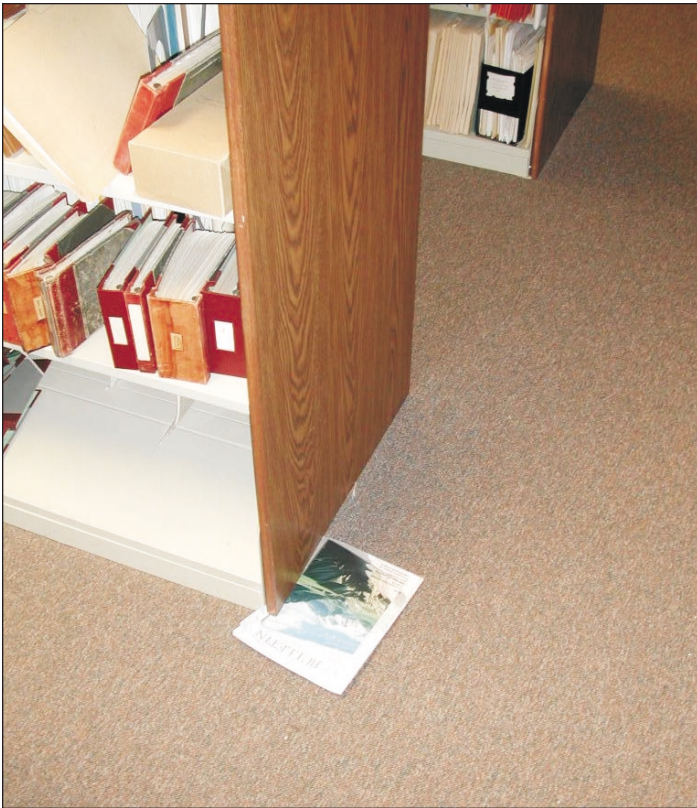
Figure 7. Proof that library shelves were lifted off the floor by the quake. Photo by Karl Wegmann.
