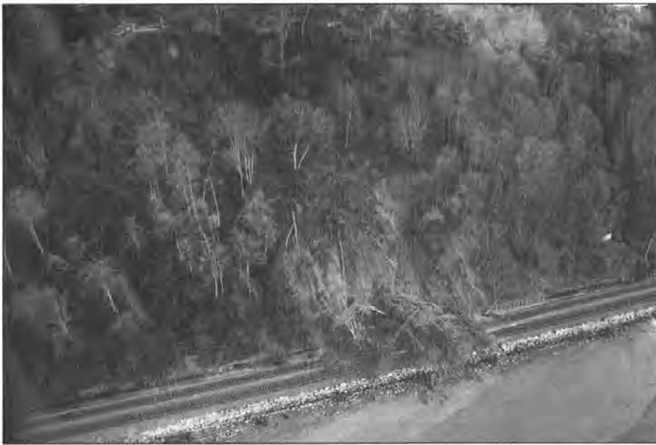
Figure 12. This slide, one of many that occurred along a stretch of railroad tracks north of Carkeek Park, lies within an older, larger slide scar. Past slides along these tracks have temporarily halted train traffic many times. Such slides have knocked railroad cars into Puget Sound, at times resulting in injuries or hazardous spills. Trip wires are strung just above the retaining wall along the tracks. An interrupted circuit signals when (but not precisely where) landslides occur. Figures 21 through 26 illustrate the different mechanisms responsible for landsliding along this stretch of bluff. Development at the top of the bluff can contribute to and is affected by the slides. Coastline modifications such as the bulkhead (built in the 1890s to support the railroad bed) also affect slope and near-shore processes. The bulkhead does not prevent landslides, but does control the rate and nature of redistribution of slide debris in the near-shore zone. Material dumped into the Sound by railroad crews cleaning the tracks is rapidly redistributed out of the narrow and steep intertidal zone and offshore by wave energy reflected off the bulkhead.
