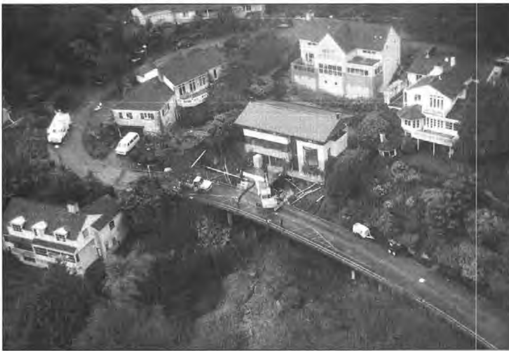
Figure 2. This house, which has been the subject of several news stories, is located on East Boston Terrace in the Capitol Hill area of Seattle. It hangs precariously over the headscarp of a reactivated old landslide. Careful construction engineering preserved the structure but not the front yard, leaving the driveway suspended. The failure of the front yard destroyed part of the road below. Note the exposed pipes, climbing ivy no longer rooted (below the tall window on the right), and tension cracks migrating into the neighbor's yard to the left in the photo. After this picture was taken, a retaining wall was built in front of the house (Seattle P-I, Feb. 6, 1997); a retaining wall behind the house was built during the original construction. This house is in the same drainage as, and a few hundred feet upslope of, a house destroyed by a landslide in 1942. That landslide killed one resident and seriously injured another.
