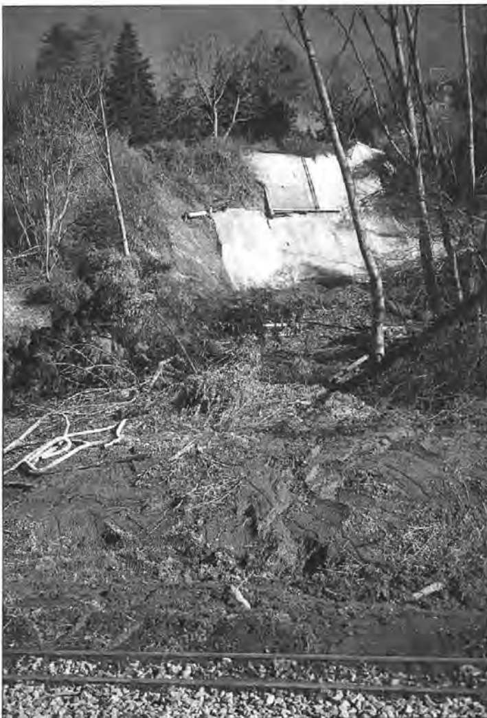
Figure 29. A resourceful homeowner in the area north of Carkeek Park, along the BNSF Railroad, used metal roofing material to cover the upper portion of the slope below his house. However, the lower part of the slope failed as a debris flow onto the railroad tracks during the December/January storms, probably because energy from runoff water was not properly dissipated, thereby causing erosion below the roofing material. Subsequently the lower slope was covered with strips from large rolls of plastic sheeting. Placing the plastic required the use of technical climbing equipment by skilled workers seen here to the left of the sheeting.
