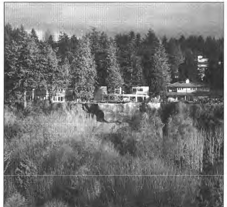
Figure 11. The owners of the house under construction in the center of this photo recognized the potential for instability at the site. The "shotcrete" (concrete sprayed on the slope) on the face of the slope was intended to protect the sandy upper part of the slope from surface erosion, but failed, probably due to excessive hydrostatic pressure. The shotcrete seems to hang like a curtain over the bluff face, with the left portion having fallen away.
