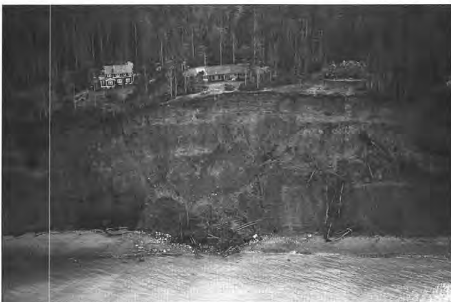
Figure 17. Fortunately, homes here were built with adequate setback—for these failures. The depth of a failure surface can influence the rate of retreat of the edge of the upland surface. In this slide west of Port Townsend, shallow debris avalanching (far left) has caused no significant edge retreat yet. The mid-bluff bench on the right indicates a relatively deep-seated slide of upper-bluff sediments only. (See Fig. 21B.) The surface of failure for the middle slide is even deeper, "daylighting" at (or below?) beach level (Fig. 21B, C), and has caused the most retreat. At many sites along the coastal bluffs, sedimentary units are not laterally continuous, and conditions can be quite different over a distance of 100 feet or less.
