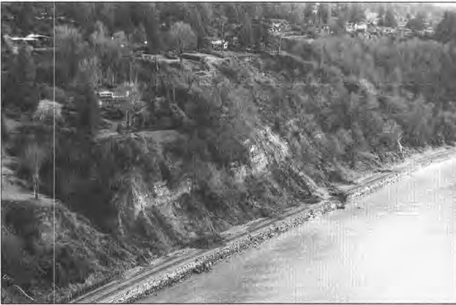
Figure 22. This view to the south shows a few of the many recent debris flows along the section of the railroad tracks north of Carkeek Park (Fig. 1). Exposed in the lower half of the bluff face are dense water-perching clays and clayey silts, which have not moved at this location. These maintain a steep bluff face that is often wet due to ground water seeping from the contact with the overlying sand. The weaker overlying sands have a much gentler slope. In the upper middle part of the photo, one can see the headscarps of older, vegetated landslides that have progressed farther back into the highlands. These features illustrate the continuing differential retreat rates of the upper and lower portions of the bluff (see Fig. 21C). The home in the left center of the photo sits in one of these landslide scars. This view shows the bulkhead that protects the toe of the slope from wave erosion (discussed in Fig. 12).
