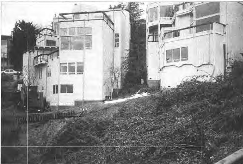
Figure 28. These two apartment buildings in the Duwamish Head area of West Seattle, just south of the intersection of Ferry Avenue and California Way SW shown in Figures 4 and 8, are built at the head of a small ravine on unconsolidated sand deposits. The February 1996 storm resulted in a shallow debris slide in that ravine. As a result, drainage from all the roofs and balconies is now collected in nonperforated pipes and directed away from the steep slope. This is called tightlining, and it is also effective along beach bluffs. There were no slides directly below these buildings as a result of the December/January storms.
