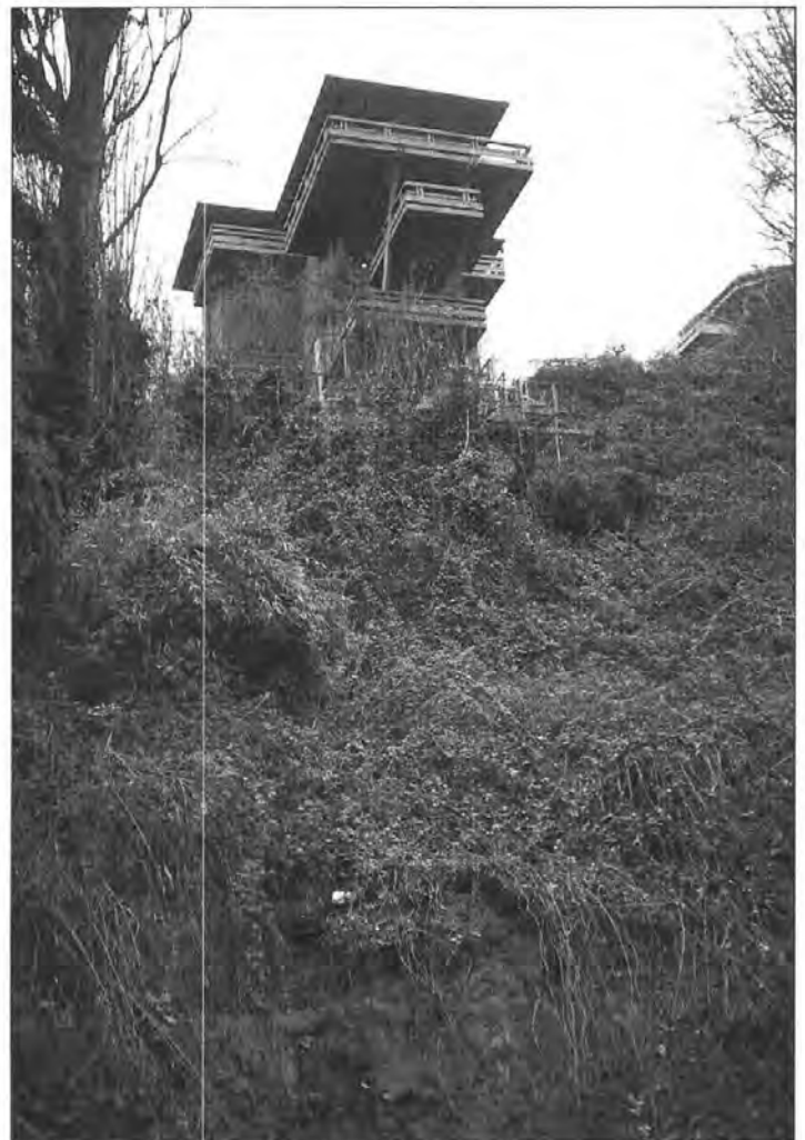
Figure 4. The "Anderson house" (known by the name of its designer) is cantilevered over the slope above Ferry Avenue SW, north of the bluff shown in Figure 3. Below it, and about 15 feet above the street, a small debris flow initiated in saturated material (here colluvium) covering clay deposits. Clay layers can be seen in the lower part of the photo. Slides like this commonly increase in size through headward erosion.
