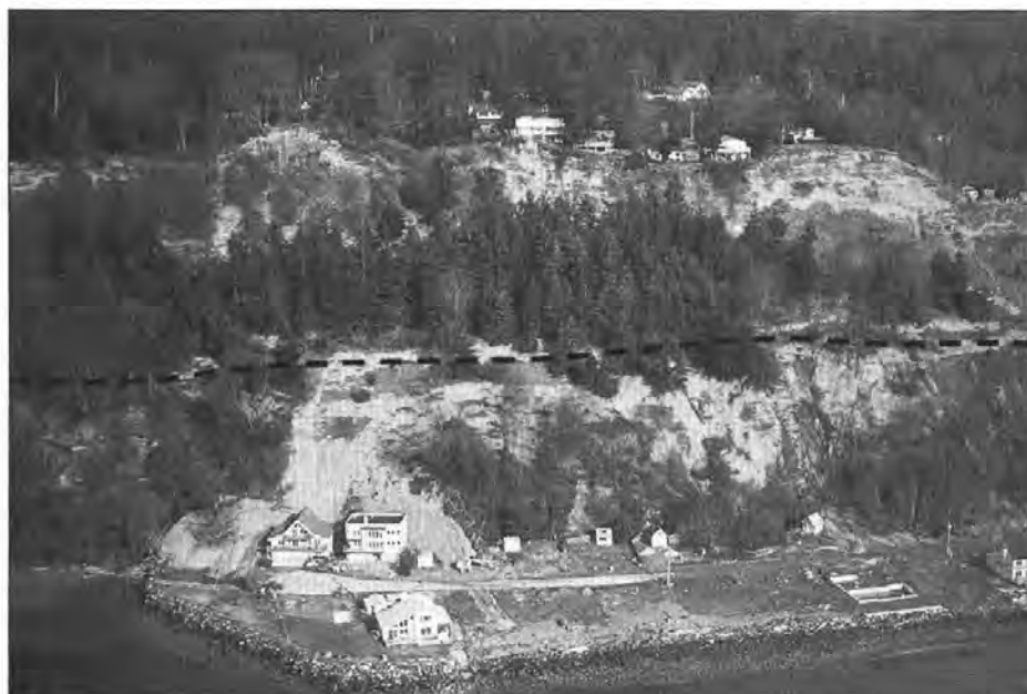
Figure 14. At Scatchet Head at the southern end of Whidbey Island, mudflows temporarily block access to these beach-level homes during wet winters. The upper bluff is porous glacial outwash sand that dries out in summer. The silt that forms the lower bluff (below dashed line) and perches ground water is damp and green year round. The top of the silt is approximately at the position of the dashed line. The scarp in the background and the partially forested bench are characteristic of such slide areas where percolating ground water is perched above the less permeable silts. The sands are weaker than the silts and slide readily when saturated. Similar situations are present north of Carkeek Park and in the Golden Gardens area of Seattle, among other places. (See Figs. 20, 21.)
