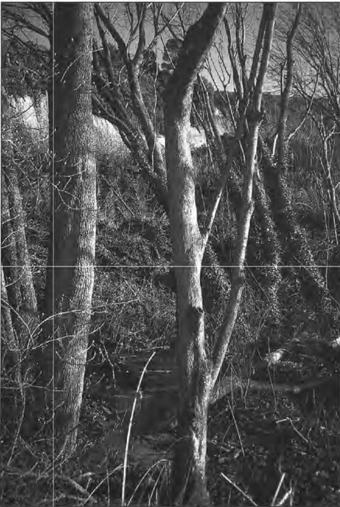
Figure 23. This view to the south (and Figs. 24–26) of the bluff along the railroad tracks (60–80 ft below) shows a fresh exposure in the Esperance Sand (Fig. 20). Shallow failures in this unit created a sand slurry (Fig. 25) that flowed onto the bench in the lower right of the photo. This location is just south of the area shown in Figure 22.
