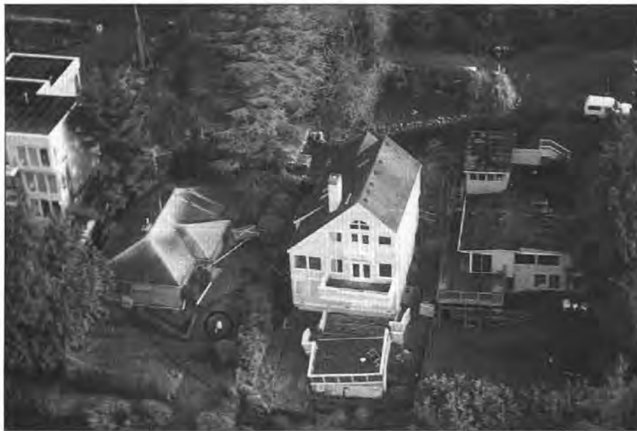
Figure 5. This view to the east shows three homes along Alki Avenue SW in West Seattle that were affected by a growing deep-seated landslide. The largest displacement occurred west (toward the viewer) of the low house on the left. Note the person (circled) standing on the down-dropped portion of the slide in front of the headscarp. Also visible is the displacement of the deck of the large house in the center. The tension crack delineating the headscarp continues through the deck area in the center house and into the backyard of the house to the right (south). The dark line extending from the house on the left is a tightline for drainage (see p. 29). Another segment of the headscarp is visible to the left of the tightline.
