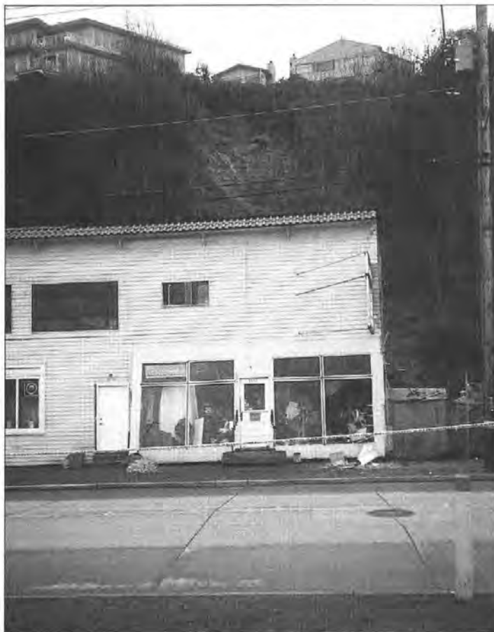
Figure 3. This boating supply store on Harbor Avenue SW stands in a line of commercial and residential structures at the base of the bluff on the east side of Duwamish Head. Many debris flows were generated along the upper portions of the bluff as a result of the December storms. At this site, a fairly small debris flow (approx. 200 yd 3 ) hit the back of the building and split into two lobes, one flowing north around the outside of the building, the other pushing through and out the front of the building. (See also the cover photo.) The area without vegetation on the bluff behind the store is a layer of sand that failed when it became saturated by ground water perched on the underlying clay. An explanation of this common geologic situation is given in Figures 20 and 21.
