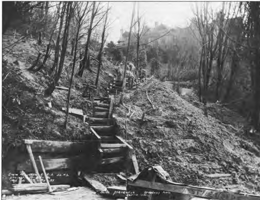
Figure 7. A slide drain trench snakes across the hillslope of the Broadway Avenue East and East Blaine Street slide (site 19, Fig. 2). (Used with permission of the Special Collections Division of the University of Washington Libraries, UWNeg#15387.)
