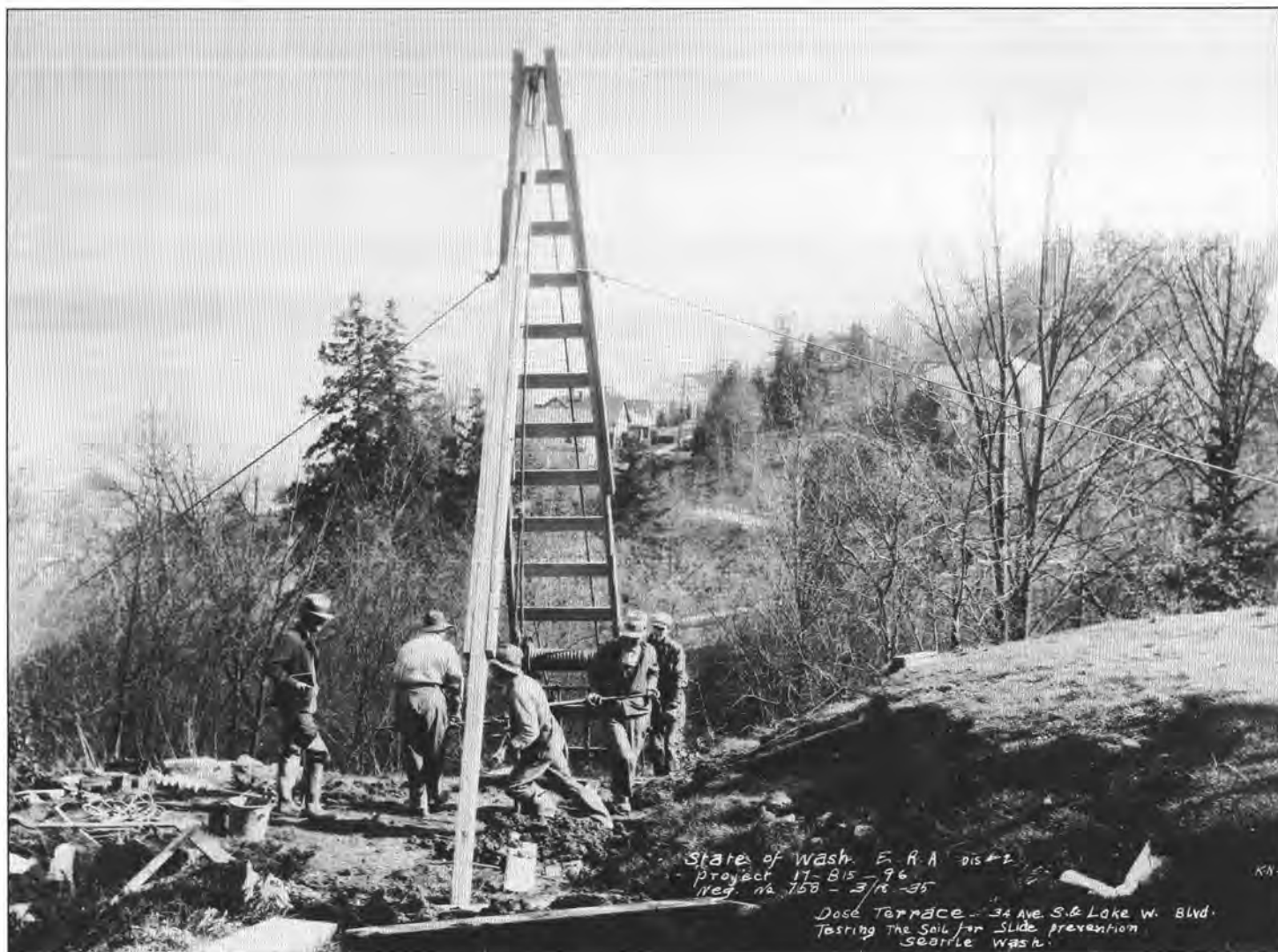
Figure 4. (See p. 7.) Hand-auger exploratory boring being drilled to test the soil for slide prevention on South Dose Terrace slide—34th Avenue South and Lake Washington Boulevard (site 22, Fig. 2). Photo taken March 16, 1935. (Used with permission of the Special Collections Division of the University of Washington Libraries, UWNeg#15388.)
