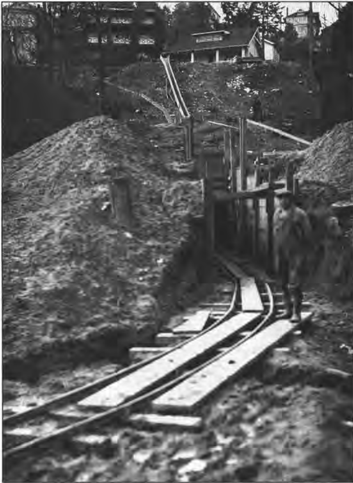
Figure 9. Slide control drain tunnel portal, Madrona Drive and East Pine Street slide (site 16, Fig. 2). (Courtesy of the City of Seattle Engineering Department.)
