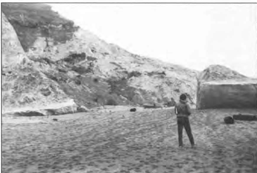
Figure 6. A walk along the bluffs of Centerville Beach south of Ferndale revealed numerous landslides, soil slumps, and rockfalls. Here the bluff (about 60 ft tall) of sands and clays failed onto the beach where much of the material was subsequently removed by waves.
