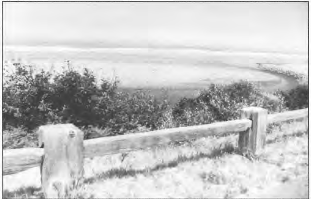
Figure 3. View west from a vista overlook on Highway 101, overlooking the mouth of the Mad River. Note the riprap along the north side (right bank) of the river. Since 1989, the river has migrated from a position just south (left) of the area shown in the photo.
