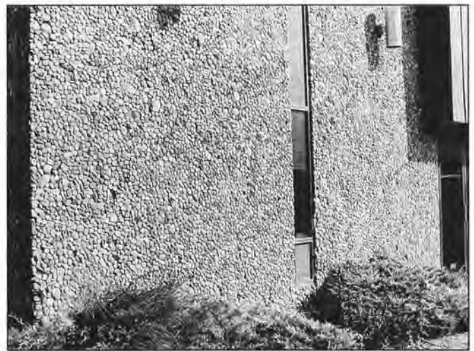
Figure 1B. Two-inch-diameter river rock aggregate is exposed on the face of these "tilt-up" prefabricated walls.
