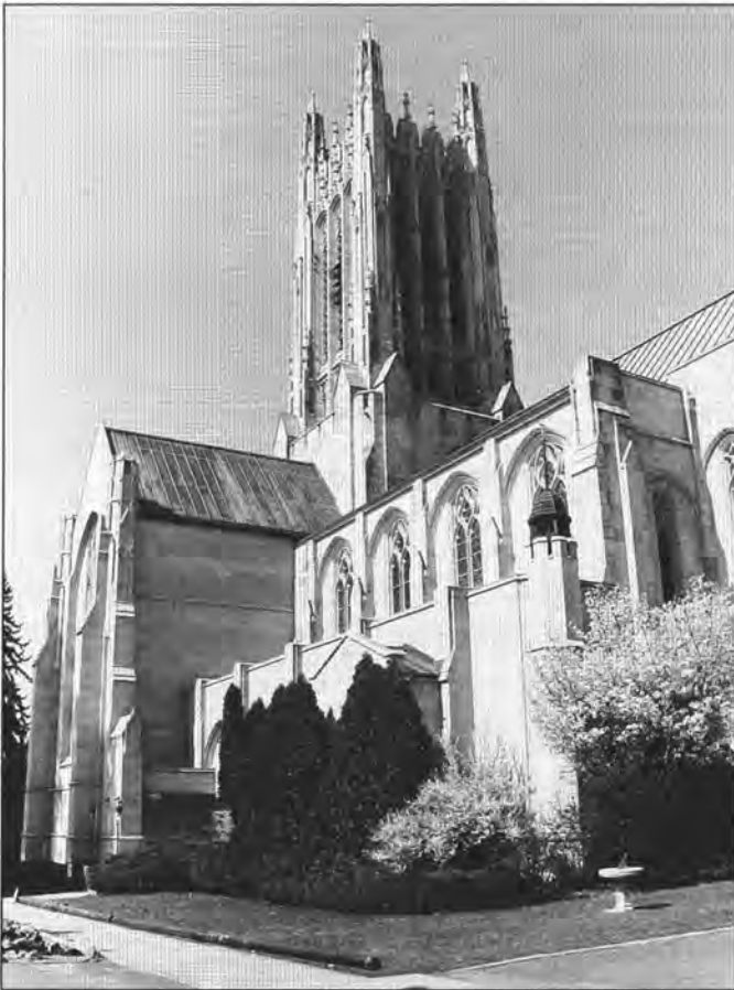
Figure 3. The exterior of the Episcopal Cathedral of St. John the Evangelist in Spokane was constructed from dimension stone cut from sandstone near Wilkeson. Each stone was cut for its particular place and was numbered accordingly. This gothic building, built in the shape of a cross, took 12½ years to complete, but there was a long hiatus before, during, and after World War II. The cathedral interior contains Boise Sandstone and Indiana limestone.
