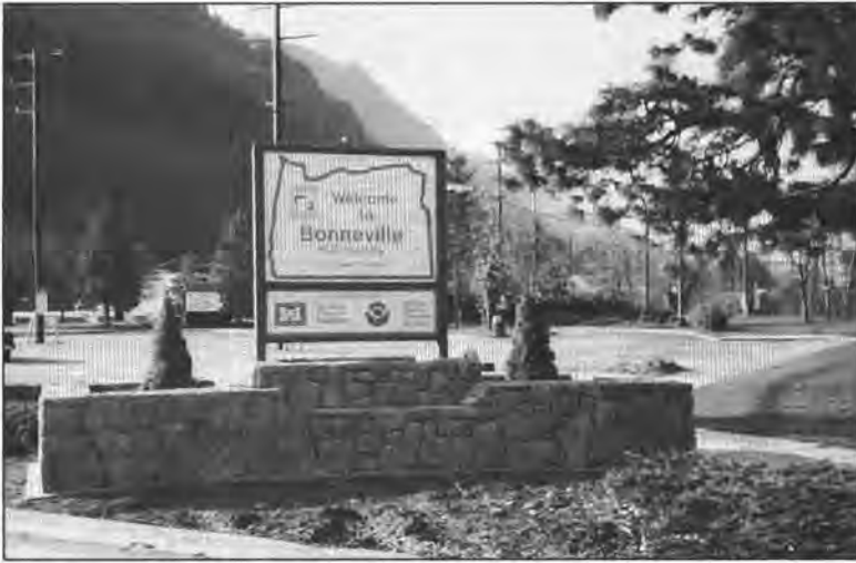
Figure 9. Camas Gray used as veneer in part of a sign. This rock is also known as Camas Gray Basalt. Photo courtesy of Tracy Lambert, Gilbert Western Corp.
