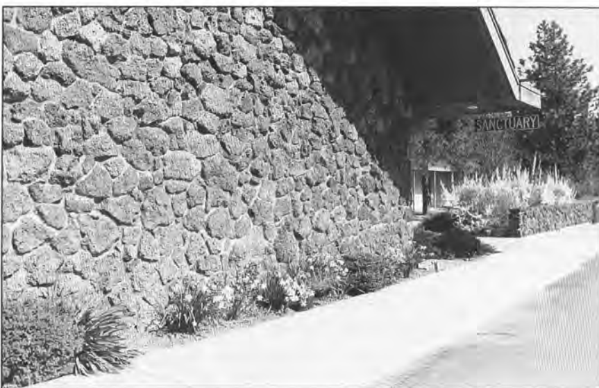
Figure 7. This mortared fieldstone wall composed of vesicular basalt boulders is an example of a common use of building stone in Washington.
