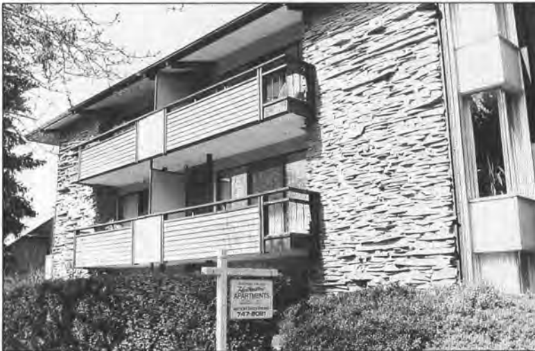
Figure 10. Andesitic "Heatherstone" forms striking ashlar walls at this apartment complex. These apartments were named for the trade name of the building stone.
