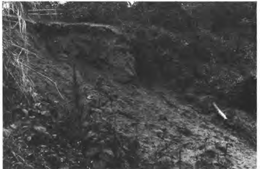
Figure 3. The headscarp of a slide crowning the top of a debris flow track. This scarp cuts the slope a scant 8 m from the foundation of a house. Failure occurred in fill material (and other debris) at the end of the yard. A drainage pipe which discharges onto the slope is visible to the right.
