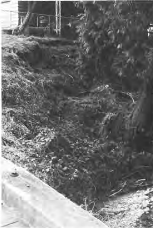
Figure 4. A slump that developed adjacent to an eroded stream channel. Here the failure threatens a house (upper left). Failures such as this can extend meters, even tens of meters, from the channel. This potential hazard should be considered when siting structures adjacent to streams.
