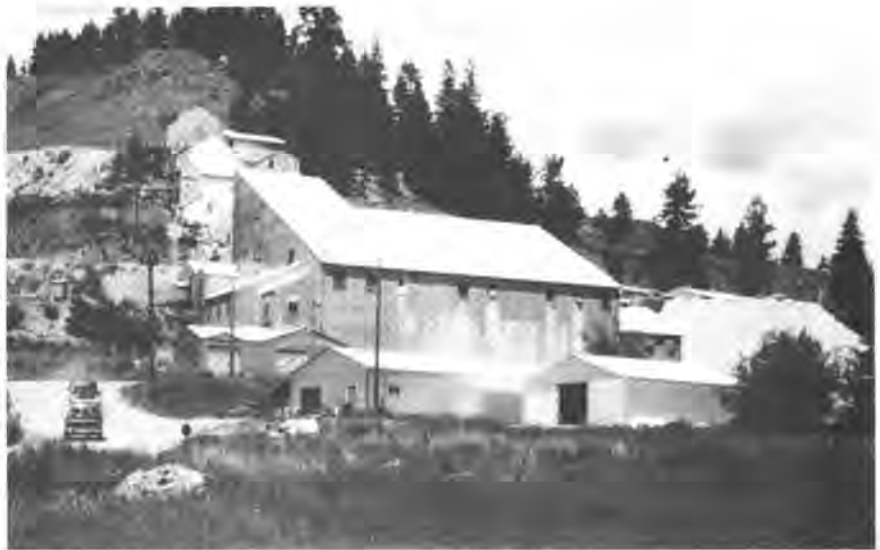
Republic Unit concentrator. Built in 1937, the mill combines flotation and cyanidation methods to recover precious metals from the ore.
