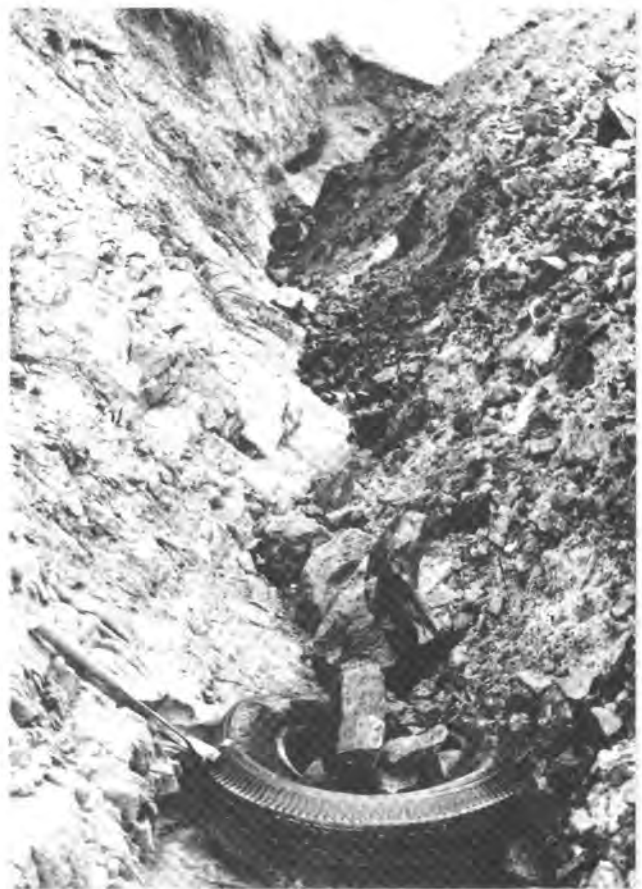
Figure 10. Landslide dam in Canyon B. The toe of the landslide is on right, scoured bedrock on the left; a tire is being crushed between the two masses, indicating continued instability.
