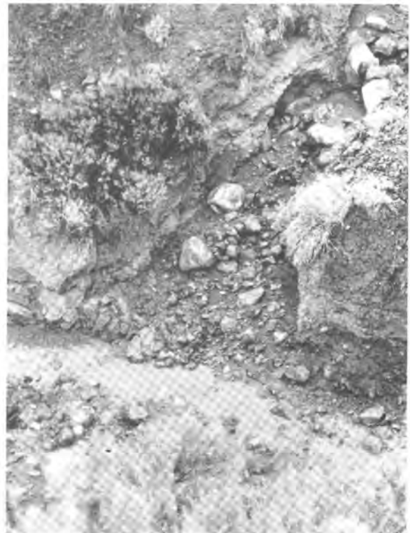
Figure 5. Confluence of a tributary and the main channel. Note the contrast between the well-armed tributary channel floor and the sand-choked main channel. Bushes are about 2 feet tall.
