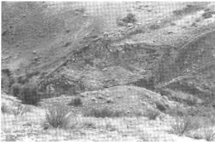
Figure 6. Reactivated portion of the deep-seated failure. View is to the northwest.
