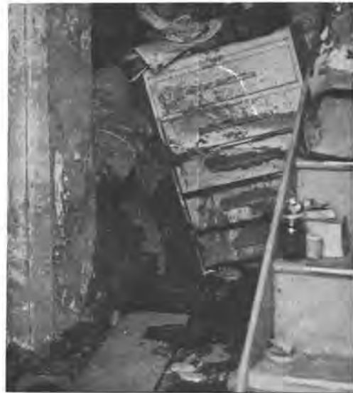
View looking in through front door of home. Mud filled lower story to a depth of several feet, collapsing floors in places.
