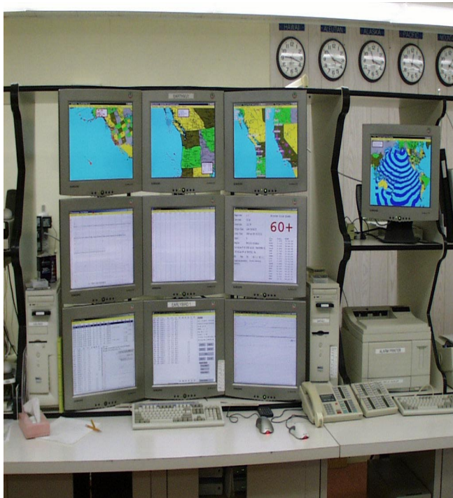
Figure 1. The Ops console. The EarthVu computer drives the top 4 screens--which show the homebrewed GIS (program written by Paul Whitmore). Displays the current earthquake location as well as selected overlays of earthquake history, tsunami history, lat/lon grid, seismic and tide instrument locations, topo contours, roads, cities, etc. The bottom 6 screens are driven by the EarlyBird computer which is used to monitor and display the realtime seismic data, analyze seismic traces and make P-time picks, compute magnitude, send messages, and basically perform the guts of the operation.
