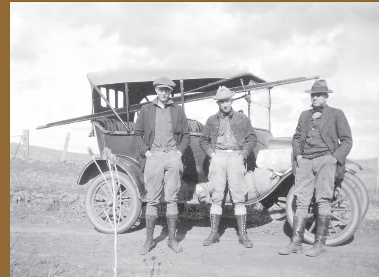
1923: Much of our early work was performing topographic surveys in cooperation with the U.S. Geological Survey
