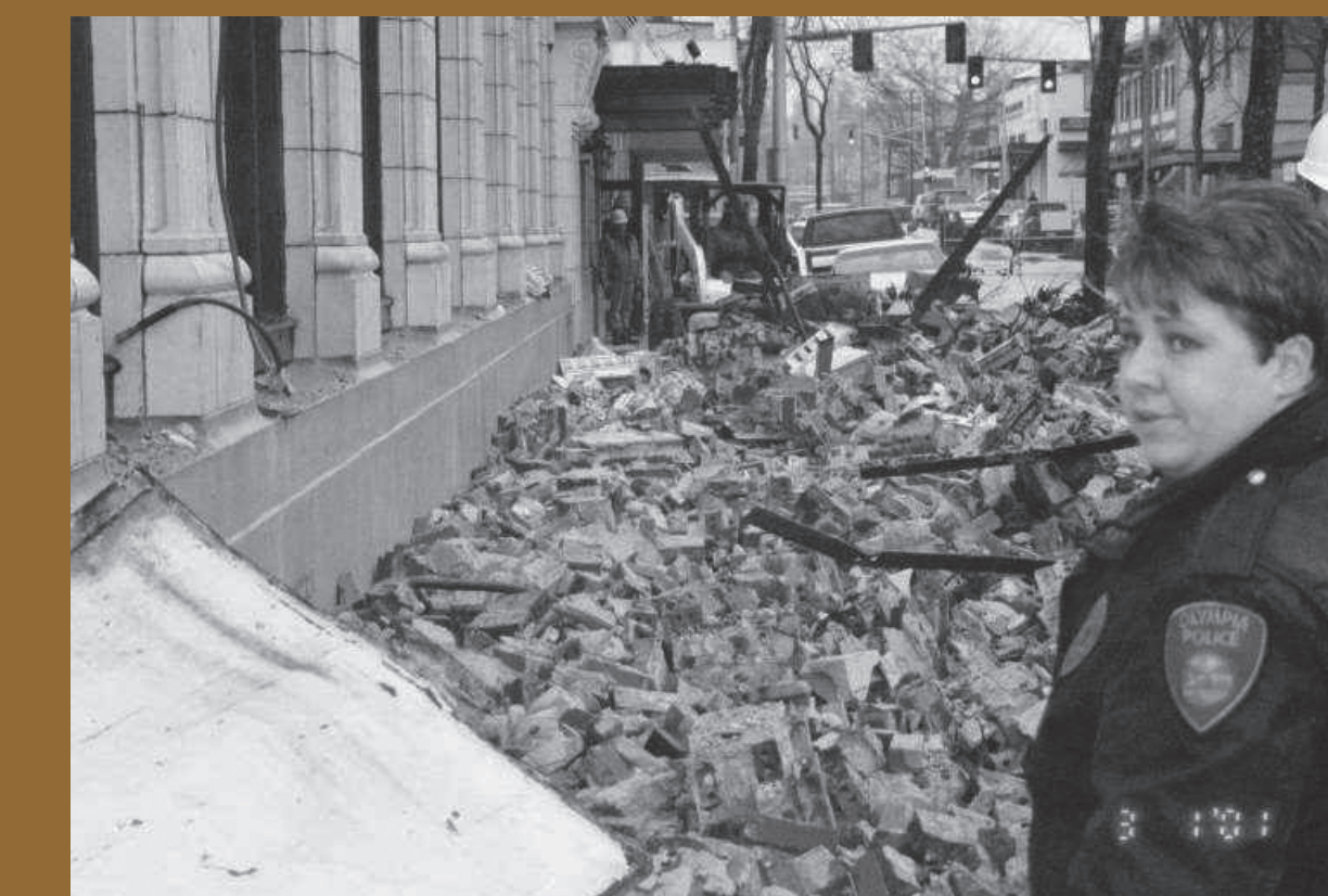
2001: Collapse of parapet of Washington Federal Savings building during Nisqually earthquake, downtown Olympia
