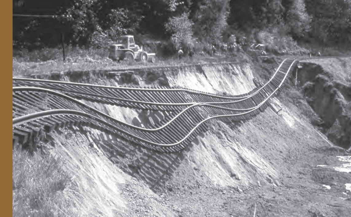
1965: Union Pacific branch rail line collapse during Puget Sound earthquake near Tumwater, Washington
