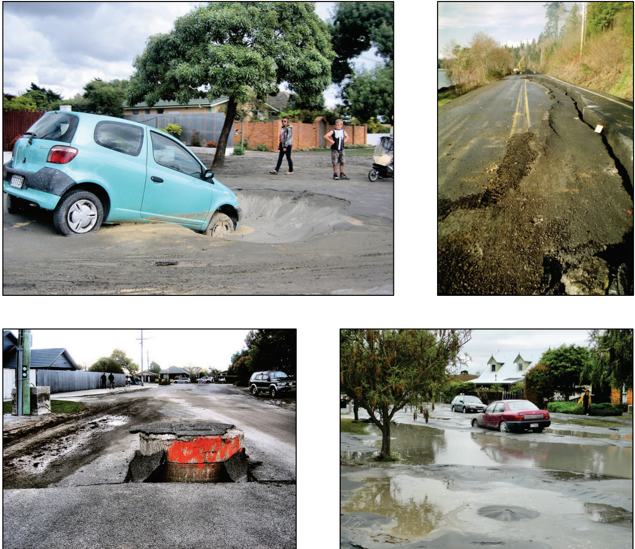
Figure 2. Examples of seismically induced liquefaction damage to transportation networks in Olympia, Wash., and Christchurch, New Zealand. Top left. A large hole created by liquefaction on a paved road during the 2011 M6.3 Christchurch, New Zealand, earthquake. The hole was likely filled with silty water resulting from liquefaction when the car drove into the hole. Note the dried water line on the side of the car. Photo: Martin Luff. Top right. Deschutes Parkway in Olympia, Wash., after the 2001 M6.8 Nisqually earthquake. Photo: Bill Lingley. Bottom left. A buoyed storm drain passes through the pavement of a road during the 2011 M6.3 Christchurch, New Zealand, earthquake. Photo: Martin Luff. Bottom right. Sand blow from liquefaction spreads sediment and water across a residential road during the 2011 M6.3 Christchurch, New Zealand, earthquake. Photo: Martin Luff.
