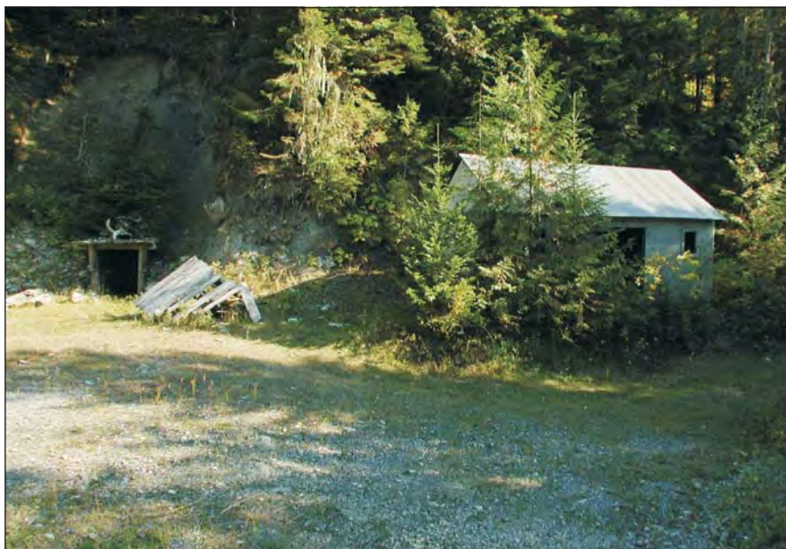
Figure 8. Mine office with main haulage adit to the left of center.
