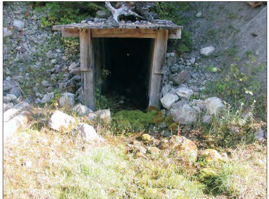
Figure 4. Main haulage adit.
