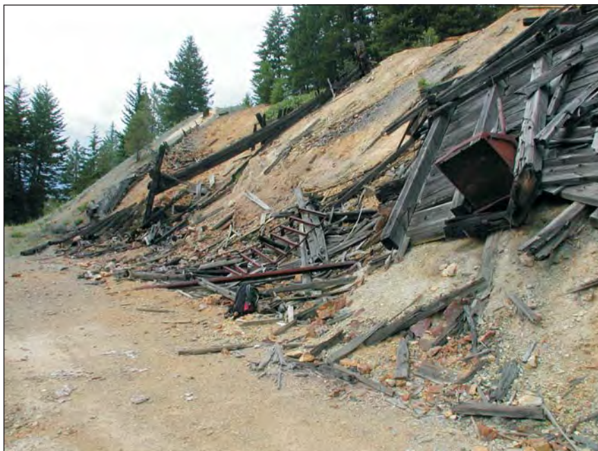
Figure 10. Remains of the ore-loading bunker. View to the north.
