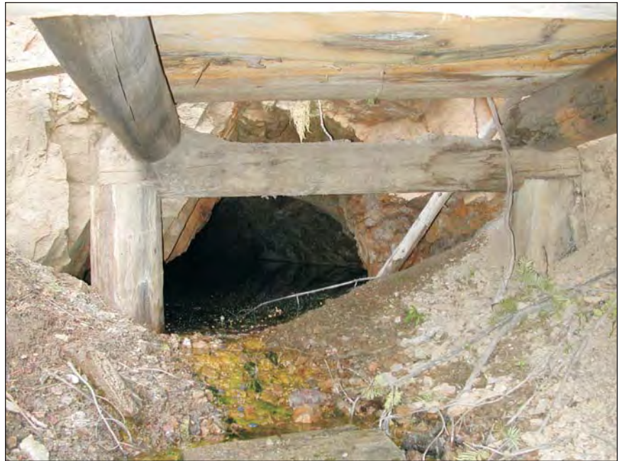
Figure 8. Entrance to level 4 (Fargo level). View to the east. Water impounded behind colluvium slough is discharging in foreground.
