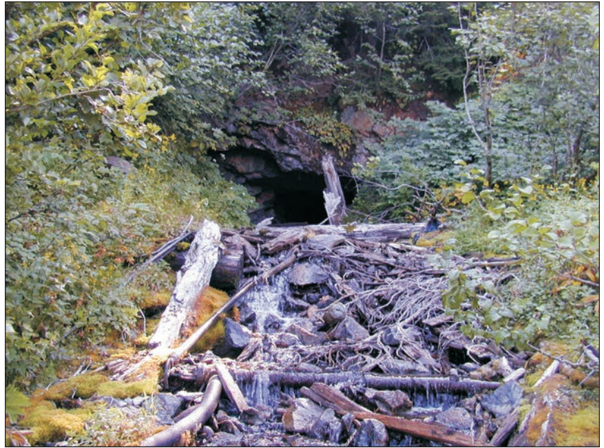
Figure 6. Water discharging from 1200 Level portal. Miscellaneous piping and mill equipment in foreground. View to the south.
