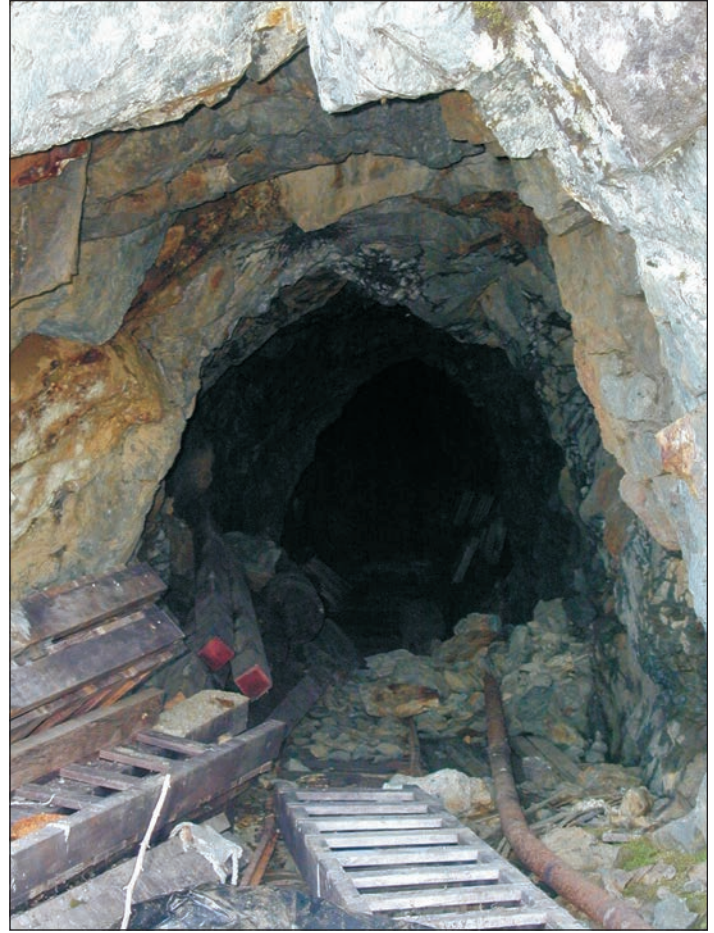
Figure 4. 500 Level portal with circa-1989 ladders and timbers.
