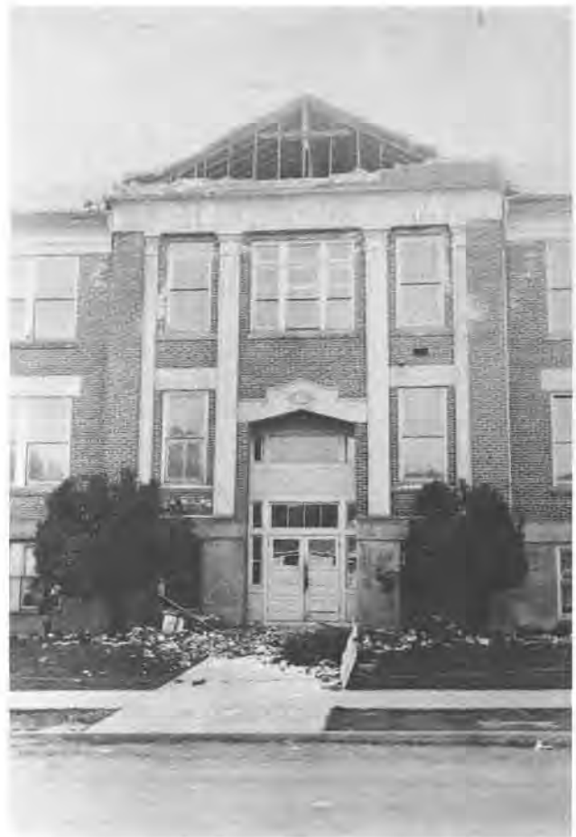
Figure 40. This unanchored gable collapsed at the Castle Rock High School in the 1949 earthquake. The building is of unreinforced masonry construction. A student was killed by falling bricks. (Photo from A. E. Miller Collection, University of Washington Archives)
