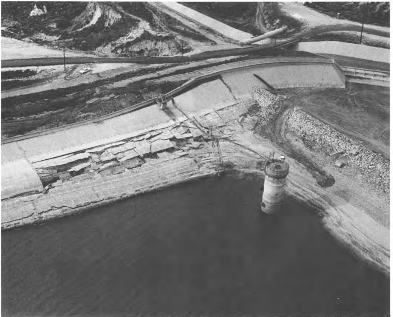
Figure 38. Damage at the Lower Van Norman Dam by the February 9, 1971, San Fernando, California, earthquake; view to the east. A massive slide into the reservoir broke off the east outlet tower and damaged the west outlet tower (foreground). No water overtopped the dam, and no leaks developed as a result of the shaking. More than 75,000 residents were evacuated from the area downstream for 3 days after the earthquake. (Photo by G. W. Thorsen)
