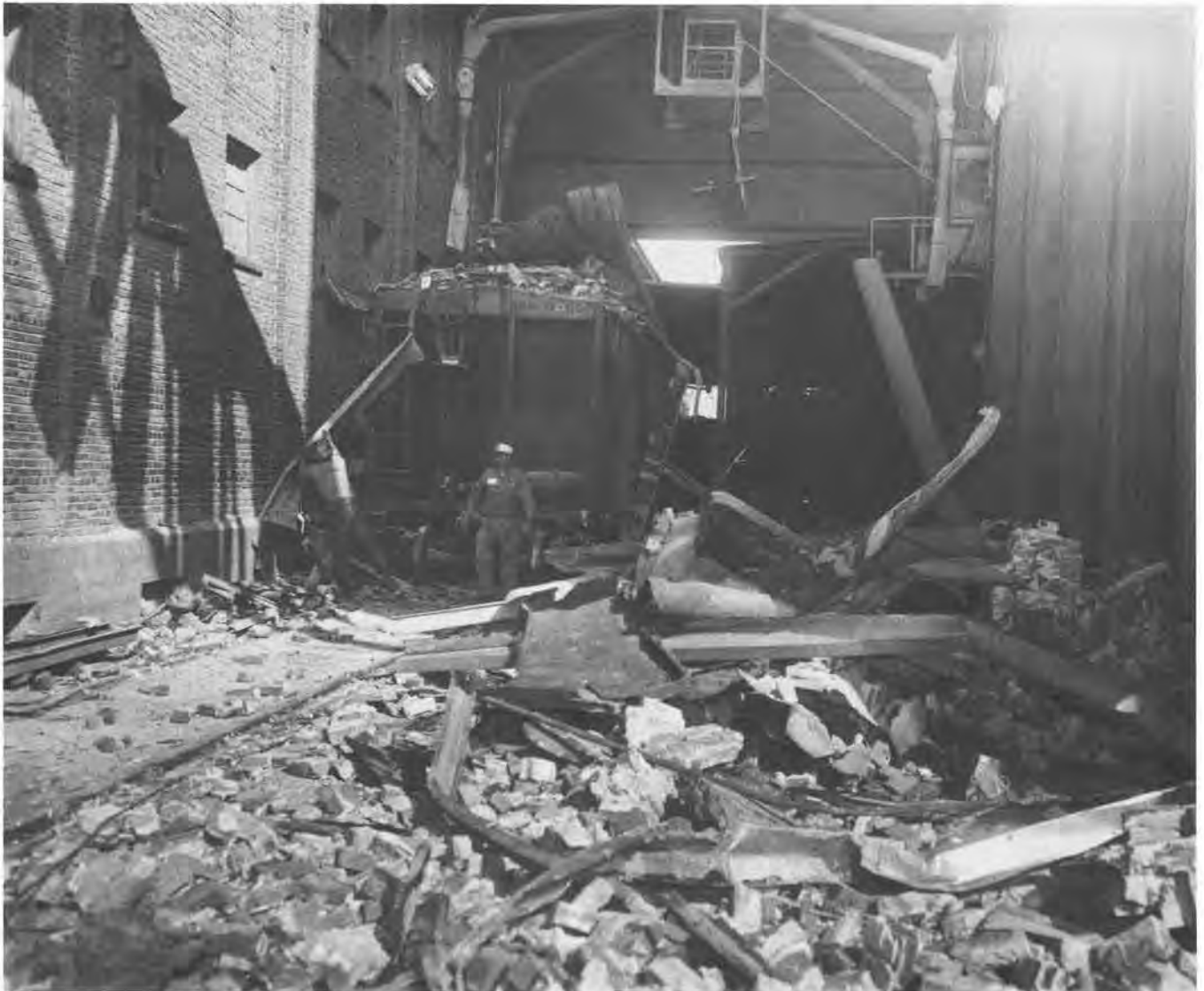
Figure 28. Portions of the unreinforced brick walls on the sixth floor of the Fisher Flouring Mills collapsed to the ground during the 1965 earthquake. (Photo by The Seattle Times Co.)
