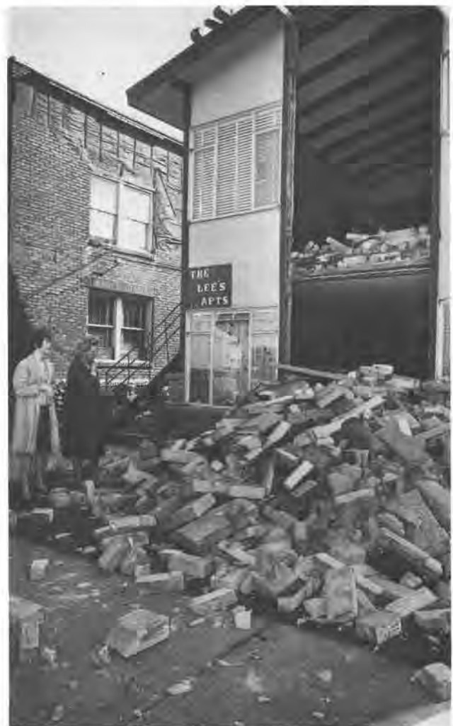
Figure 27. Failure of unreinforced masonry used in a Seattle apartment building. Damage was caused by the 1965 earthquake. Note that the wood frame part of the building was undamaged. (Photo by The Seattle Times Co.)
