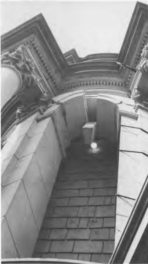
Figure 43. An unanchored keystone in an arch in the Capitol Building dome loosened by ground shaking in the 1949 Olympia earthquake. (Photo from the A. E. Miller Collection, University of Washington Archives)
