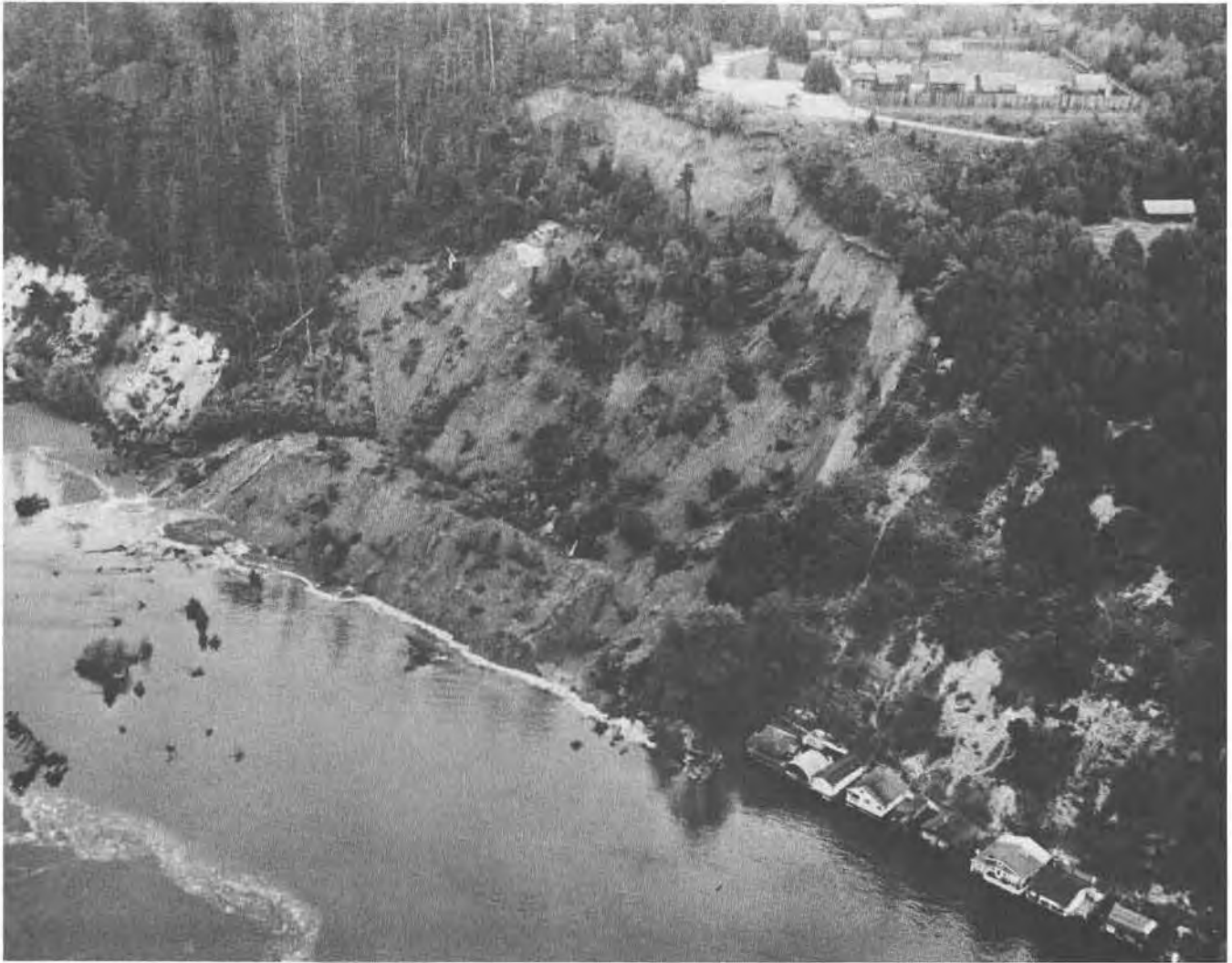
Figure 20. This ground failure was initiated by ground cracking adjacent to the banks of the Tacoma Narrows during the 1949 Olympia earthquake; the slide occurred several days after the earthquake. The landslide endangered nearby homes and induced strong waves in the Narrows. (By permission of Wide World Photos, Inc., and Associated Press)
