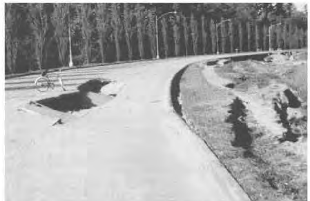
Figure 21. A road in Olympia that was damaged in 1965 by liquefaction. (Photos by G. W. Thorsen)
