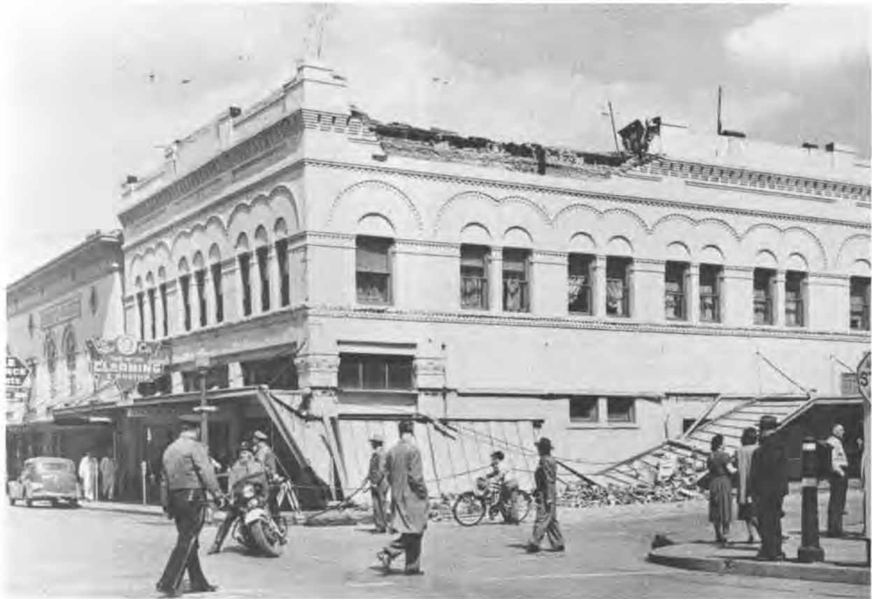
Figure 30. A collapsed parapet wall and crushed canopy in downtown Olympia, 1949 earthquake. (Photo by Roger Easton, by permission Marie Cameron)
