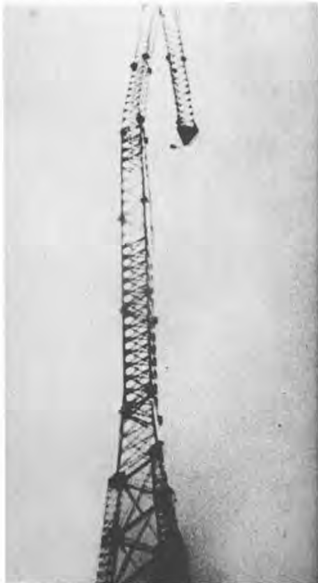
Figure 37. Damage to the tower of Seattle radio station KJR caused by the 1949 Olympia earthquake. (Photo from A. E. Miller Collection, University of Washington Archives)
