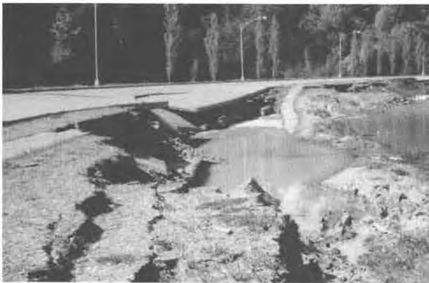
Figure 21. A road in Olympia that was damaged in 1965 by liquefaction. (Photos by G. W. Thorsen)
