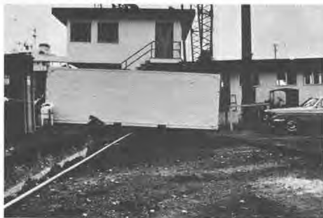
Figure 39. The ground at this Harbor Island, Seattle, site dropped when the pier at the left shifted toward the water in the 1965 earthquake. (Photo by K. V. Steinbrugge, from Steinbrugge and Cloud, 1965)
