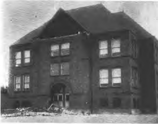
Figure 41. Lafayette School in Seattle after the 1949 earthquake. The gable fell because of lack of adequate anchorage and defective masonry. The masonry fell on the landing in front of the main entrance. (Photo from an article by C. N. Dirlam reproduced in Thorsen, 1986)
