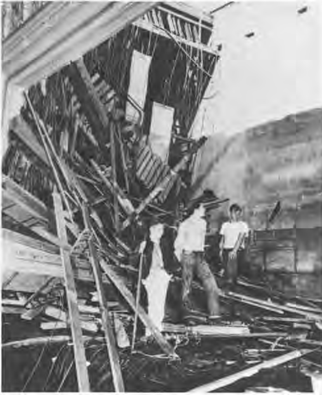
Figure 29. The unanchored roof of the Puyallup High School gymnasium collapsed onto the stage during the 1949 Olympia earthquake. (Photo by The Seattle Times Co.)
