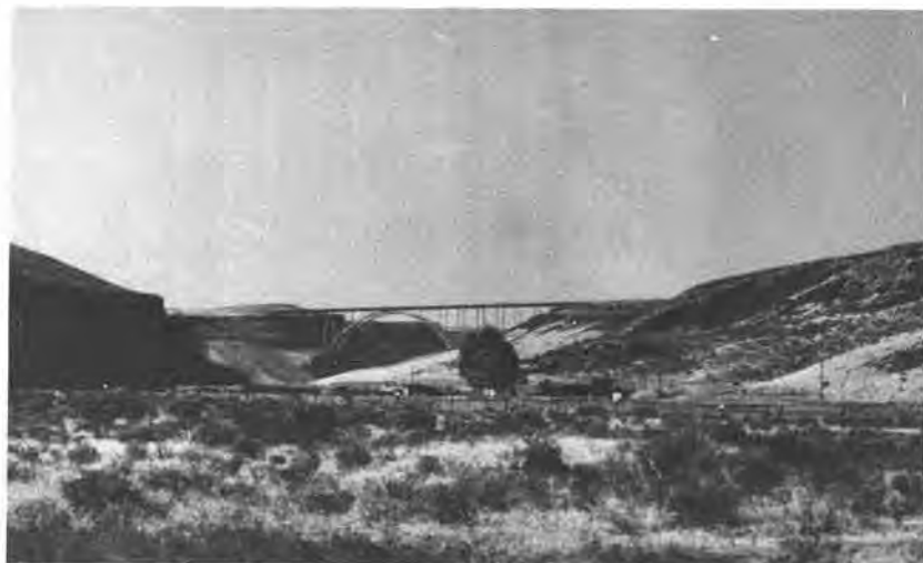
MILEAGE 24.9—Selah Creek Bridge, looking east up Selah Creek.
