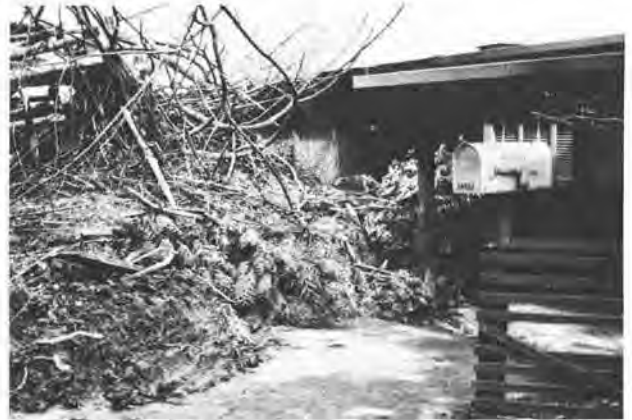
FIGURE 2.—Landslide along Edgewater Lane N.E.
