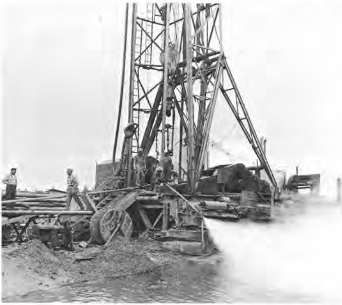
Testing of the Sunshine Mining Company-Medina No. 1 oil well, near Ocean City, Grays Harbor County. The spray coming from the pipe is a mixture of crude oil and natural gas. Figure 49.
