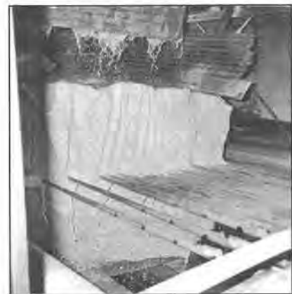
The Wilkeson stone quarry near Wilkeson, in Pierce County. Upper photo shows the working face of the quarry; note the man in the lower right-hand corner of the picture. Lower picture shows a large block of sandstone being cut by a gang saw. Figure 44.
