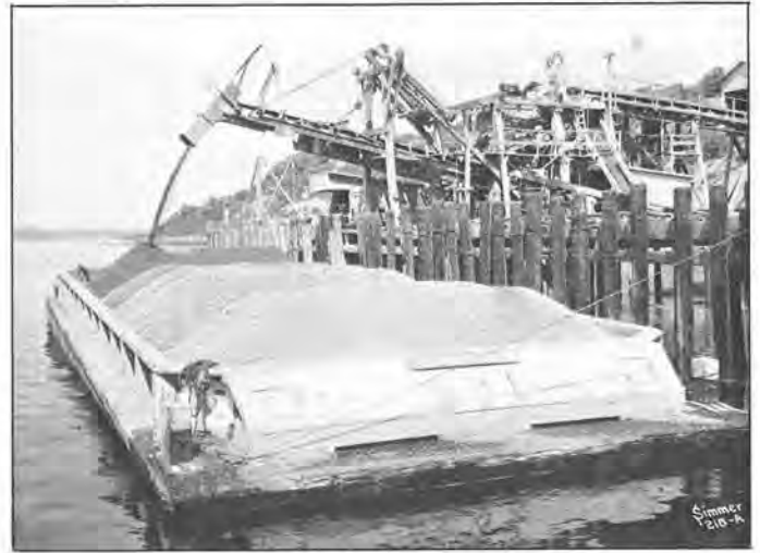
Gravel being loaded on a barge at Pioneer Sand and Gravel Company's Steilacoom gravel pit. Sand and gravel is shipped to several places around Puget Sound that do not have local sources of good gravel. (Photo by Simmer.) Figure 43.
