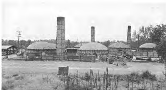
Old-fashioned beehive-like downdraft brick kilns formerly operated at Granger, in Yakima County. Most modern brick plants use continuously fired tunnel kilns to produce bricks. (Photo by Simmer.) Figure 38.
