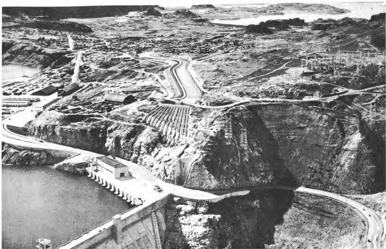
Figure 4. Upper Grand Coulee, viewed from the north, above Coulee Dam. Feeder canal, center, equalizing reservoir (floor of Grand Coulee, background). The floor of the Coulee and the foundation of the dam are granite; the walls of the Coulee are of Columbia River basalt.
