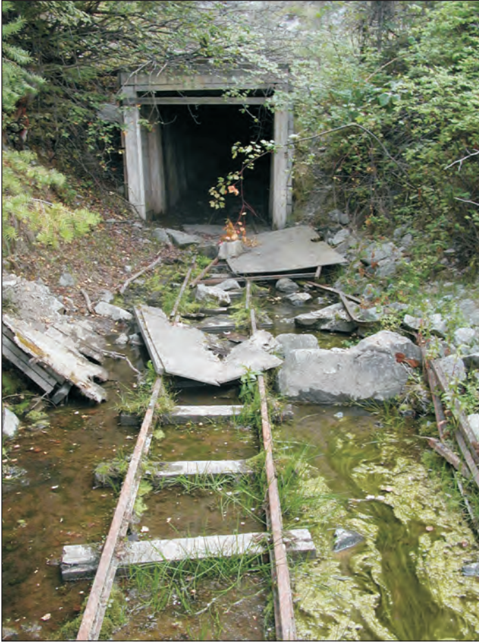
Figure 3. Lower adit portal. View to the southwest (S65°W).
