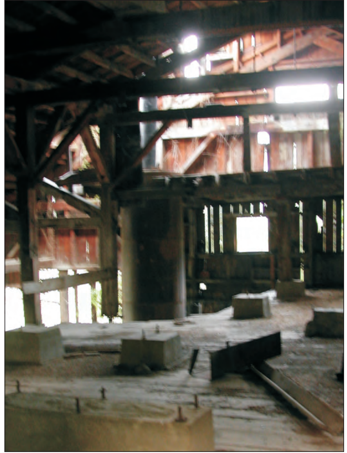
Figure 4. Mill building interior with footings.
