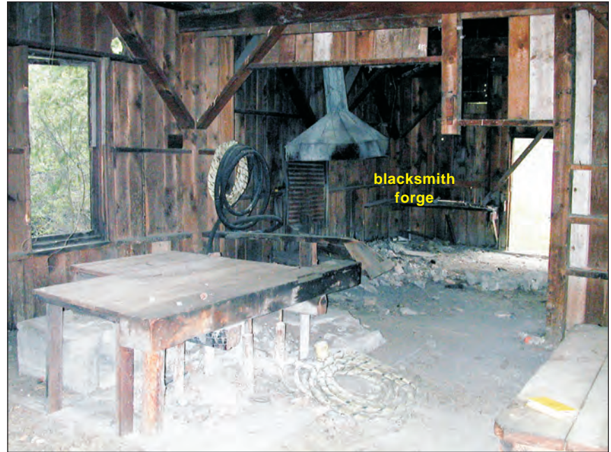
Figure 5. Interior of maintenance shop.
