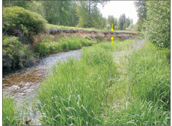
Figure 14. Cut bank on Toroda Creek. Light brown tailings (between arrows) overlie the original land surface. Flow is right to left. View is to the south.
