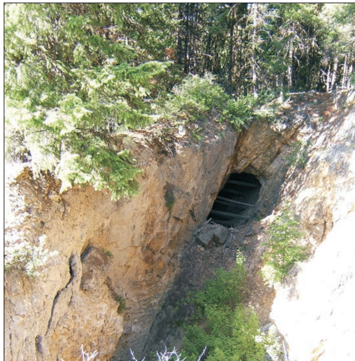
Figure 8. Open stopes along mine ridge. View is to the northeast.
