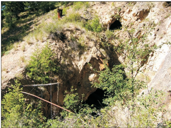
Figure 7. Open stopes along mine ridge. View is to the northeast.
