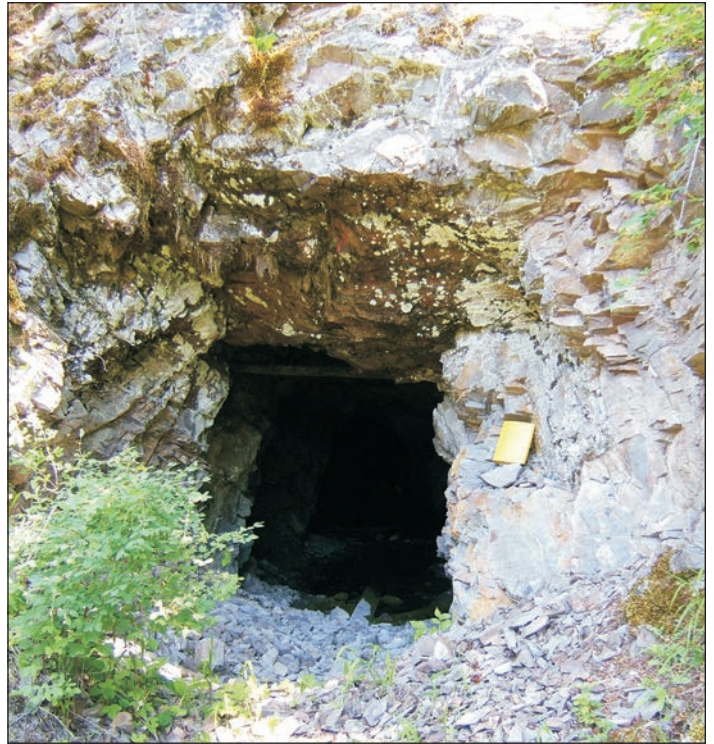
Figure 2. Massive andesite exposure at the 700-level portal. Platy fragments are spalling around opening. View is to the east.
