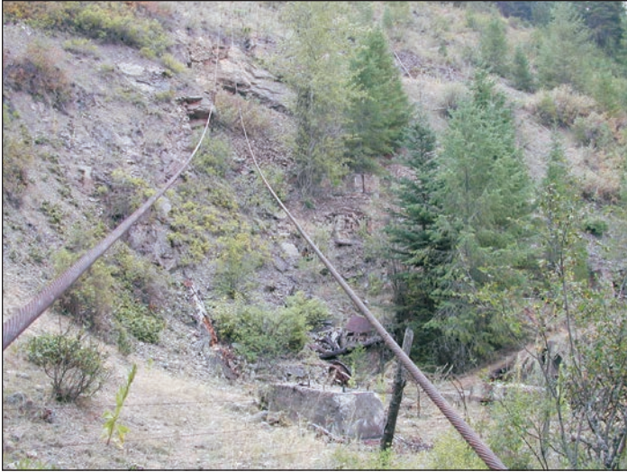
Figure 13. Mill site footing and tram cable to the 400-level adit. View is to the east.
