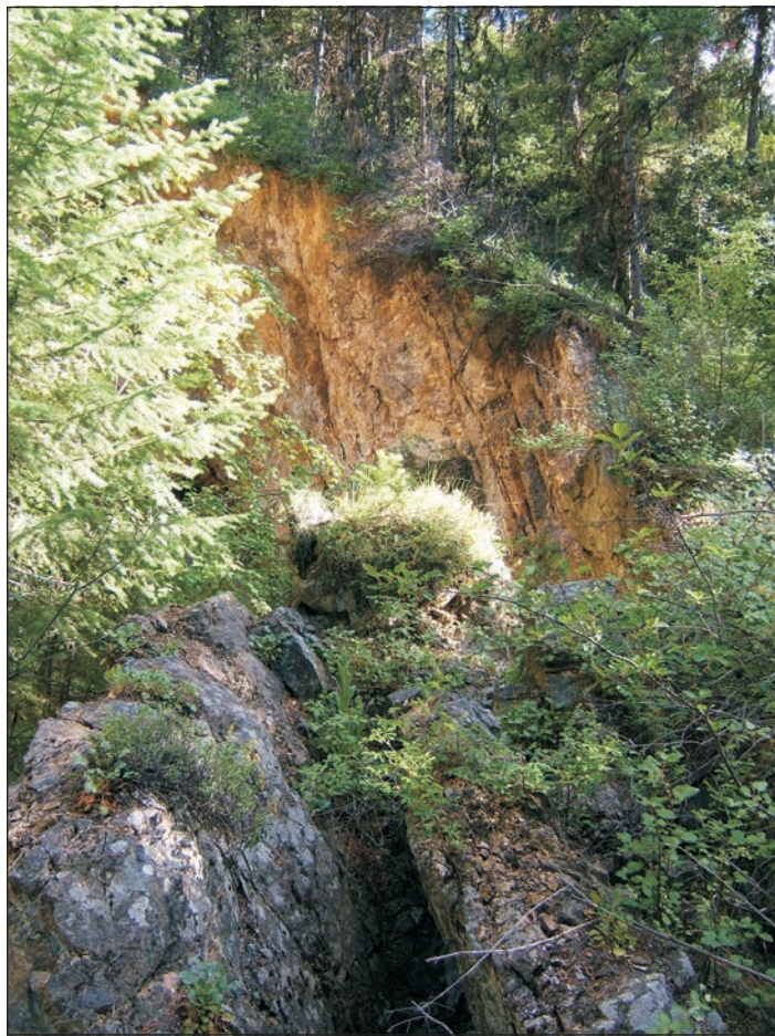
Figure 11. Ten-foot-deep cracks in the open pit hanging wall. Material is collapsing into the pit. View is to the south.
