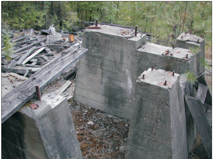
Figure 9. Mill ruins and crusher foundations.
