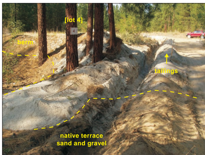
Figure 12. Real estate development utility trench through tailings. View is to the north.
