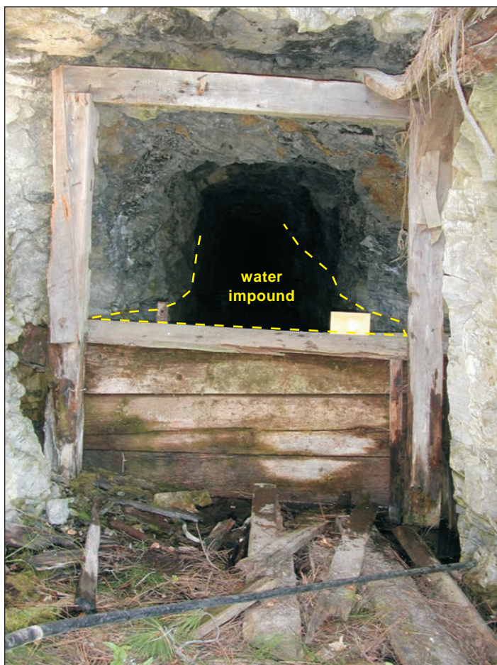
Figure 10. Water impounded behind weir at No. 1 level portal. View is to the east.
