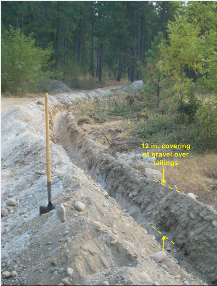
Figure 13. Tailings underlying gravel covering in trench. View is to the south.
