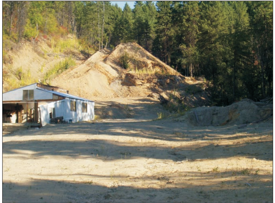
Figure 4. Gold recovery processing shed sitting on tailings from original mill. Bulldozed waste rock dump left center. View to the north.
