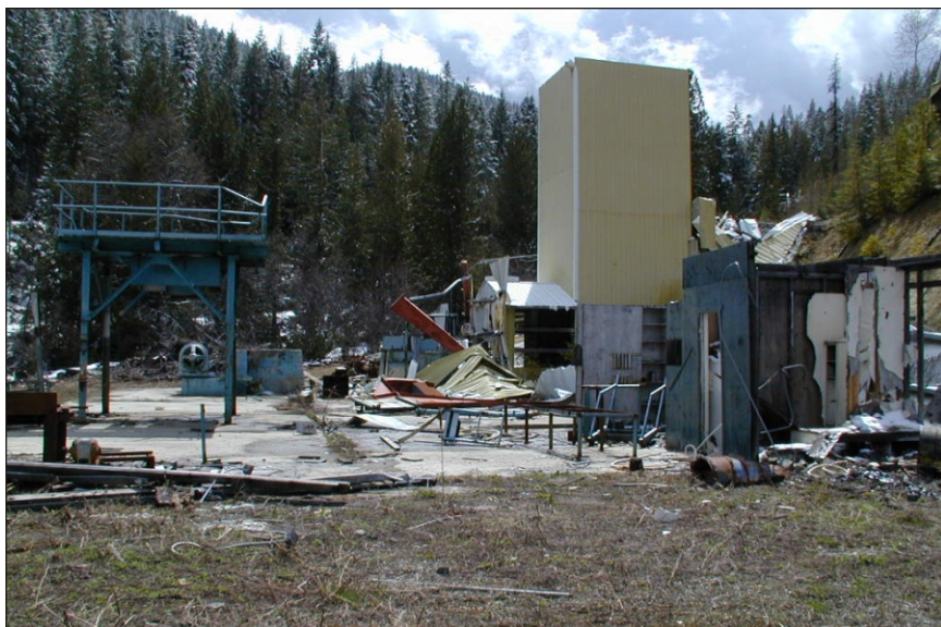
Figure 10. Remains of Madre mill site after 1988 salvage operation.
