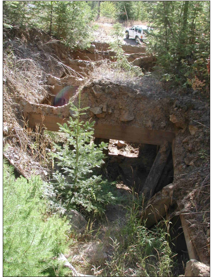
Figure 8. Exposed drift sets of the Madre tunnel. View to the east away from the adit.
