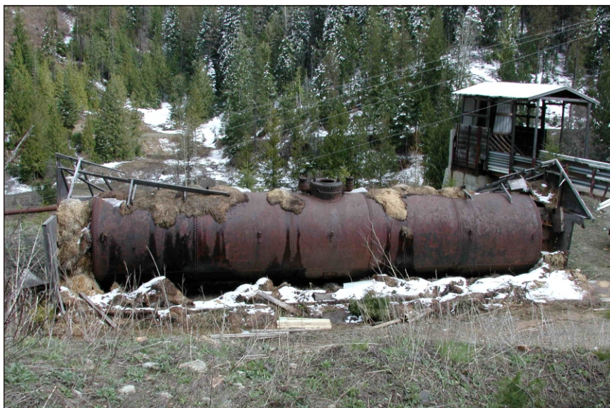
Figure 12. 15,000 gallon water storage tank. Rock tipple at far right. View to the east.
