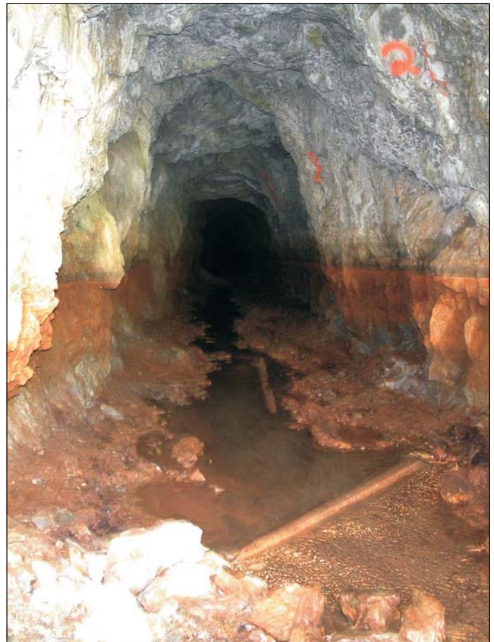
Figure 9. Water discharge at the Lower level adit. Note the iron staining on the wall to a height of about 36 inches.
