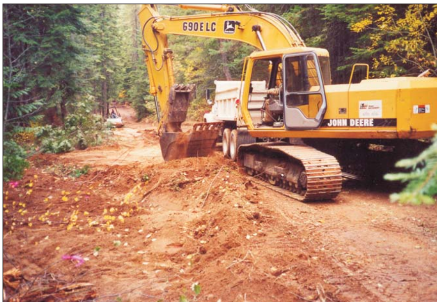
Figure 19. Excavation of tailings from mine access road on public land. View to the west. BLM photo taken October 2001.
