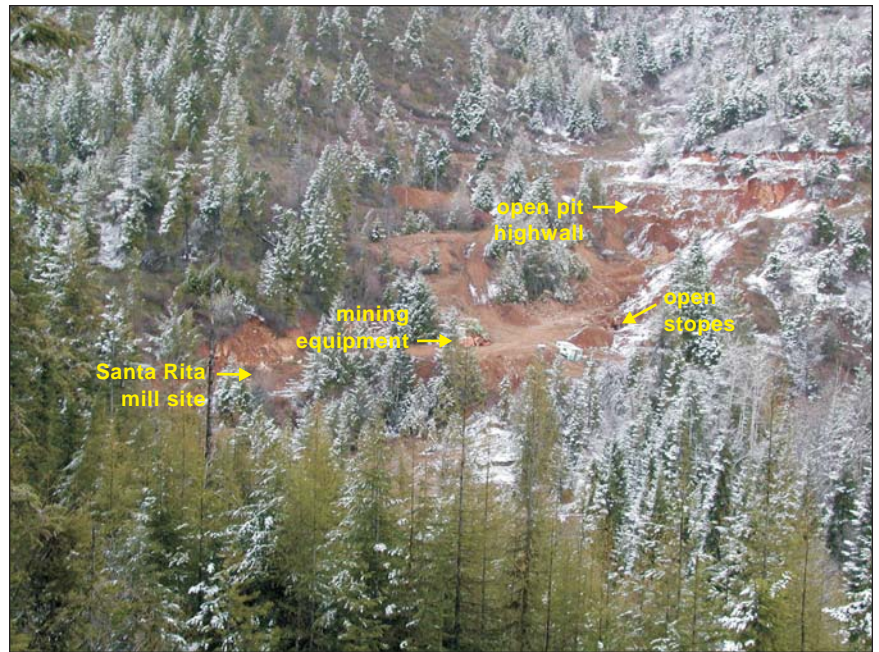
Figure 2. Partial overview of the Cleveland mine site. The Lower Level portal, tailings, and access road are off the photo at the far left center. View to the northwest.
