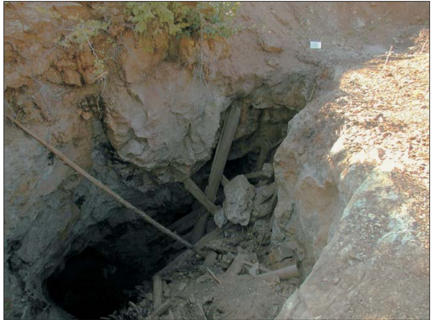
Figure 4. Underground opening excavated by surface mining. View to the southeast.
