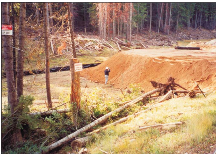
Figure 20. Roadside tailings placed in new cell adjacent to tailings repository 4. View to the southwest. BLM photo taken October 2001.
