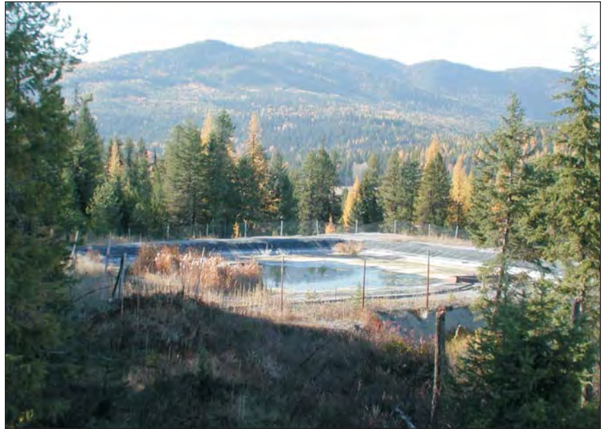
Figure 27. Waste-water retention facility near the Lower tailings pond. View to the southwest.
