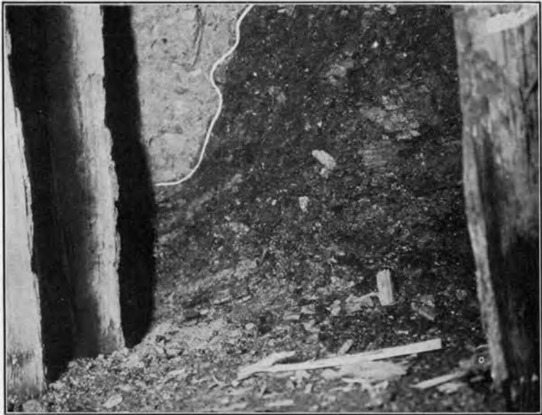
B. Beekman No. 2 Mine, Roslyn Fuel Co. Erosion of Coal and Gravel Filling Near Outcrop in Big Dirty Bed.
