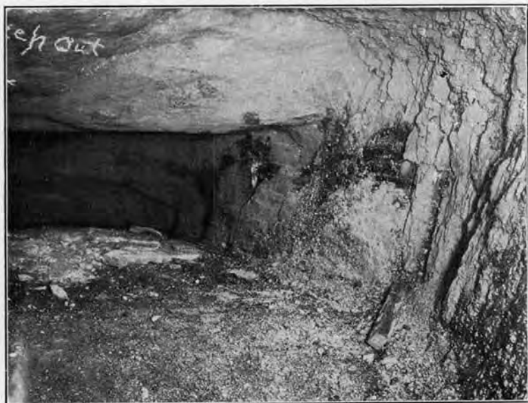
B. No. 2 Mine, Roslyn-Cascade Coal Co. Roll in Roof and Floor of Slope.
