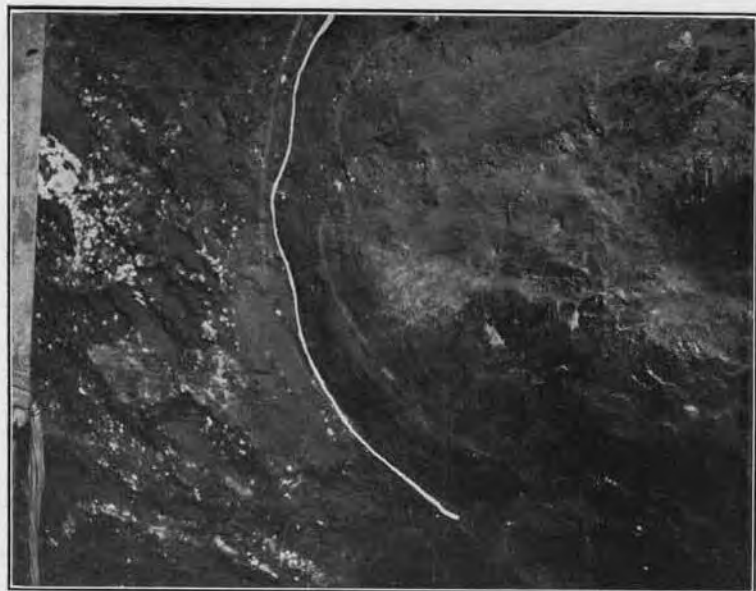
A. No. 2 Mine Roslyn-Cascade Coal Co. Roll in Roof on Main Slope Below 6th Level.
