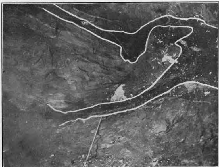
B. No. 3 Mine, N. W. I. Co. Fifth Level East on Air Course, Showing Pinching in Coal Below Rock in Photo Above.
