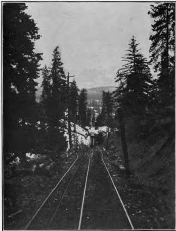
A. Parting at Center of Tram, No. 1 Mine, Roslyn Cascade Coal Co.
