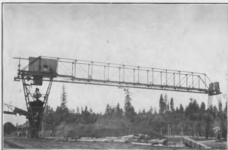
A. Conveying, Loading and Discharging System at Clealum.
