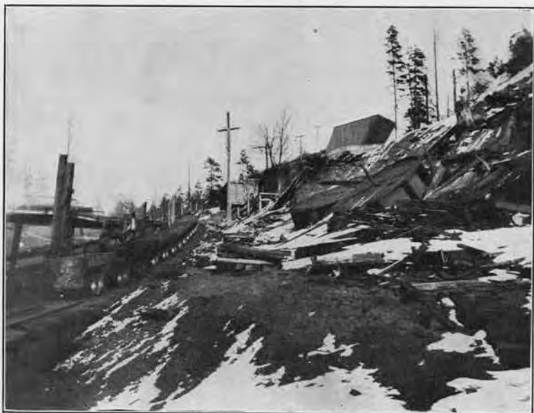
B. Looking up the Incline to No. 6 Mine, N. W. I. Co.
