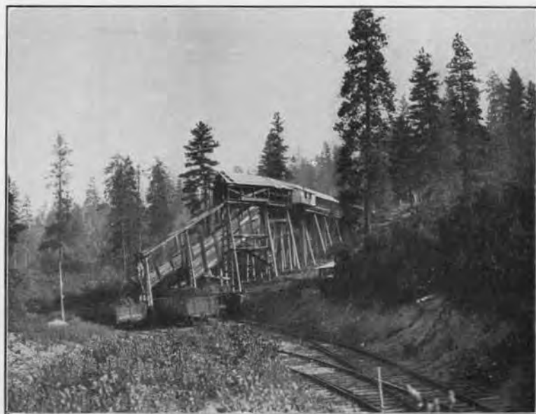
B. Tipple, showing Gravity Screens, No. 1 Mine, Roslyn Cascade Coal Co.
