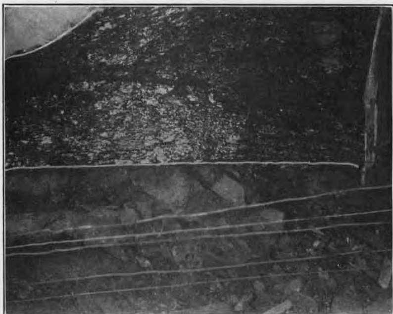
A. No. 4 Mine, N. W. I. Co. Thinning of Coal Along the Main Slope Between 13th and 14th Levels.
