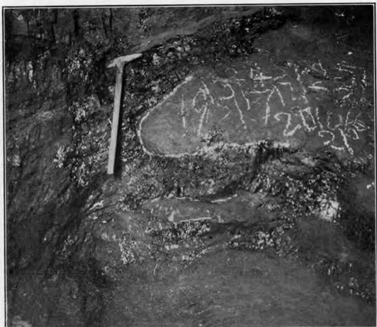
A. No. 3 Mine, N. W. I. Co. Fifth Level East, Showing Roll in Bottom and Horses of Rock in Coal.
