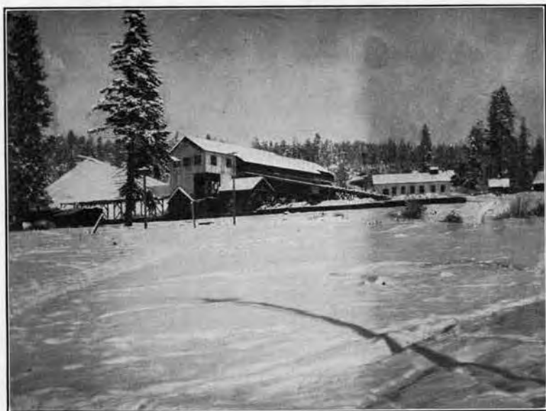
B. Tipple and Rock Dump, No. 3 Mine, N. W. I. Co.
