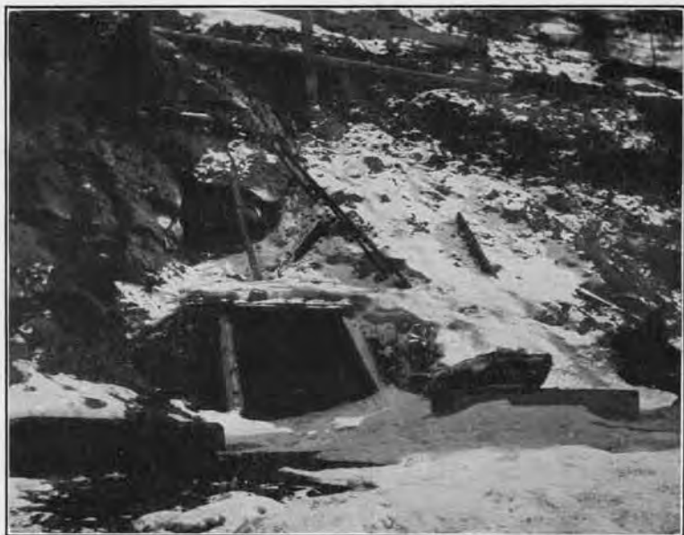
A. Drift into Hillside Just Above Original Opening to Coal. No. 1 Mine, N. W. I. Co.
