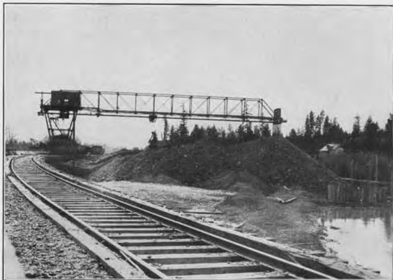
B. Storage Yard, with Conveyor, at Clealum.
