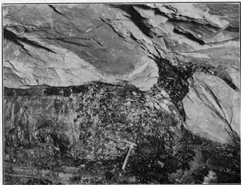
B. No. 5 Mine, N. W. I. Co. Detail Photograph Showing the Coal Squeezed Into Opening in Sandstone Roof Rock at Same Point as Above.
