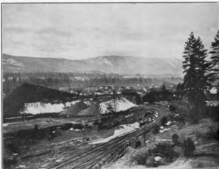
B. Clealum, Looking Southwest Across the Yakima Valley, Clealum Mine in the Foreground.
