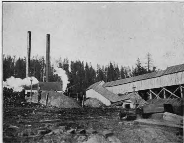
A. Power Plant and Tipple, No. 1 Mine, Roslyn Fuel Co.
