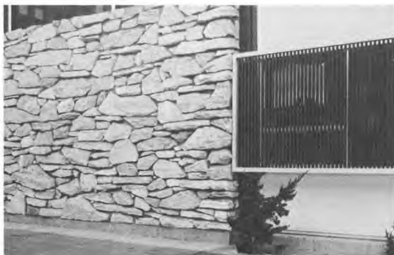
FIGURE 3.—Rough building stone wall. Note how recessed mortar accentuates the shape of the fragments of gneiss.
