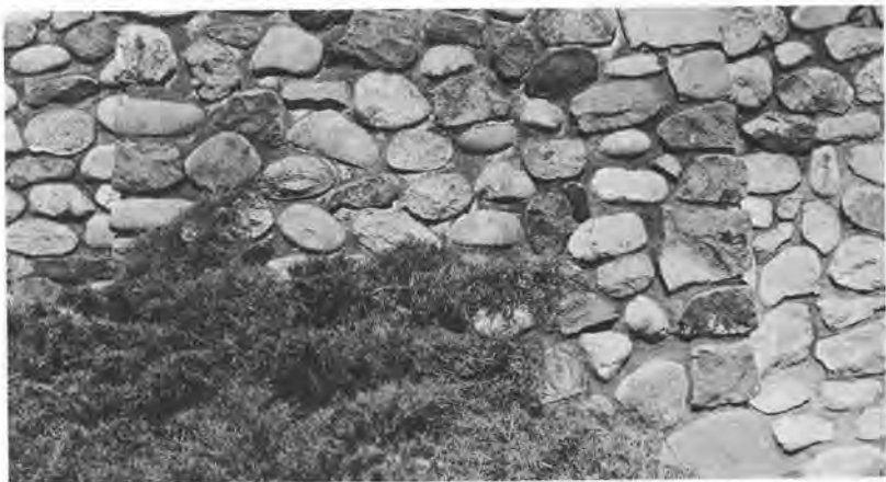
FIGURE 2.— Field stone wall, constructed from stream-worn cobbles and boulders.
