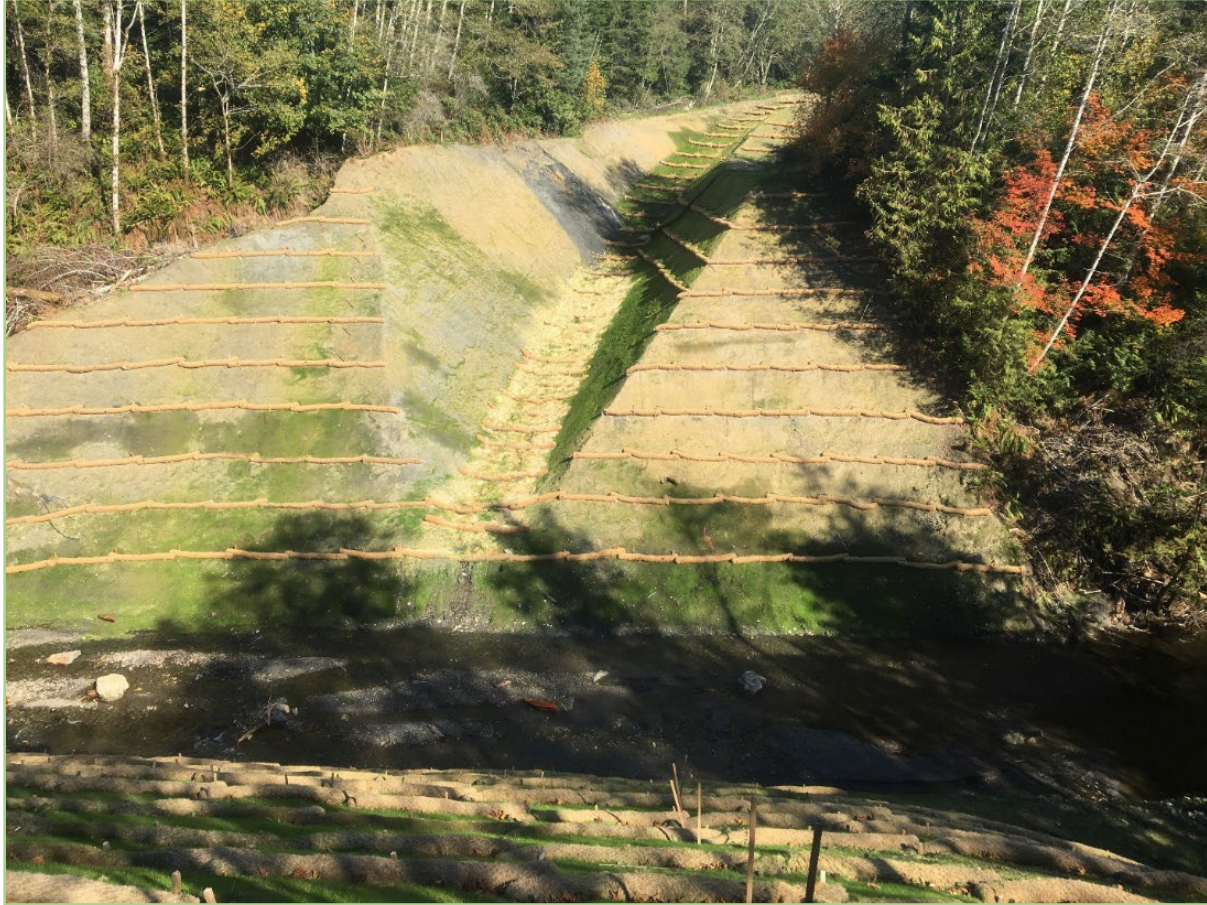
This photo is from the Crescent Unit in Olympic Region and shows bank stabilization efforts on a large fish barrier removal.
