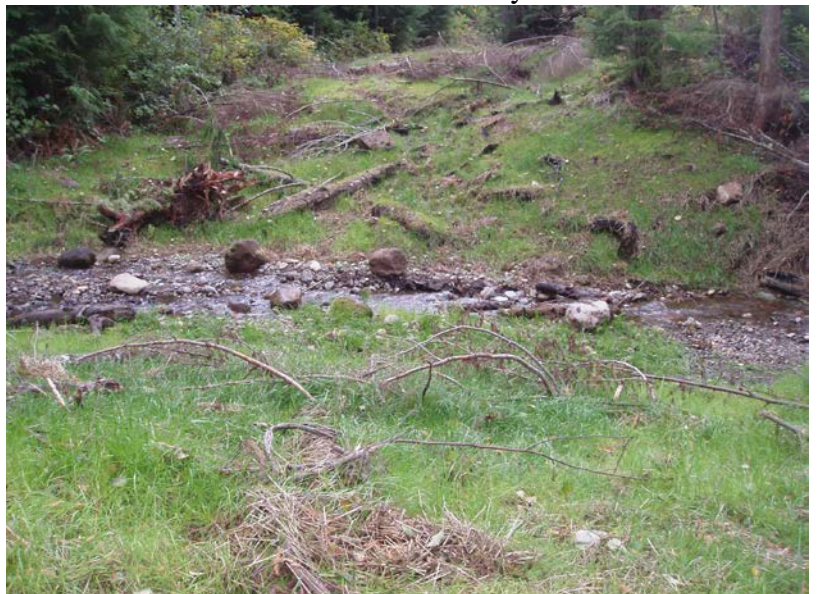
Properly abandoned road crossing
