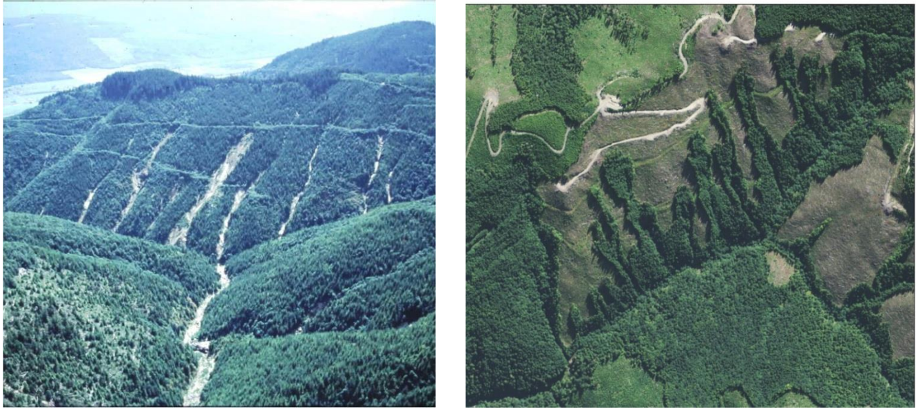
Figure 4. Left: Road-initiated debris flows in unstable landforms, Sygitowicz Creek, Whatcom County (Photo: DNR 1983). Right: Same hillslope 28 years later (2011 aerial photo).
