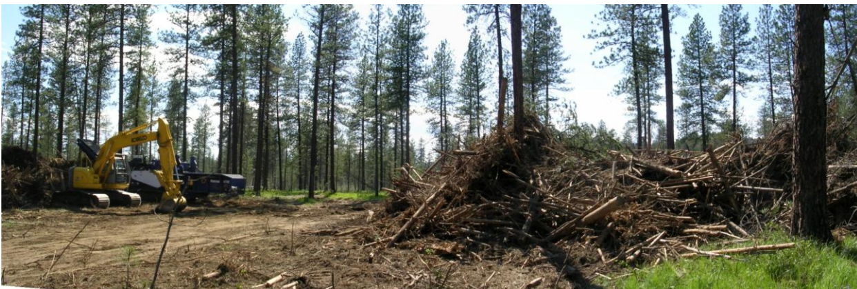
Figure 19. Processing equipment waiting for the trucks to return
