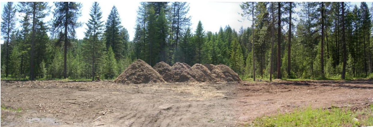
Figure 20. Slash ground and waiting for transportation to the biomass facility
