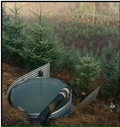
589 590 591 Figure 2: A sediment trap installed below a road segment. 592
