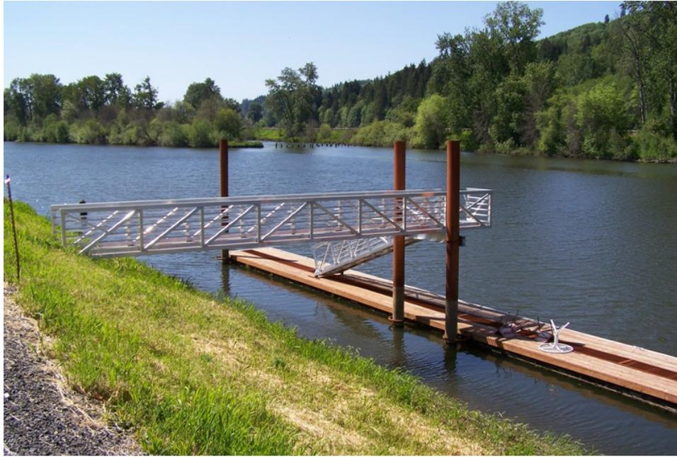
Figure 3.17 Dock with a float, pier, and gangway on the Cowlitz River. Photo: Washington DNR
