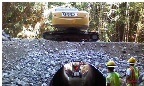
Culvert Replacement
