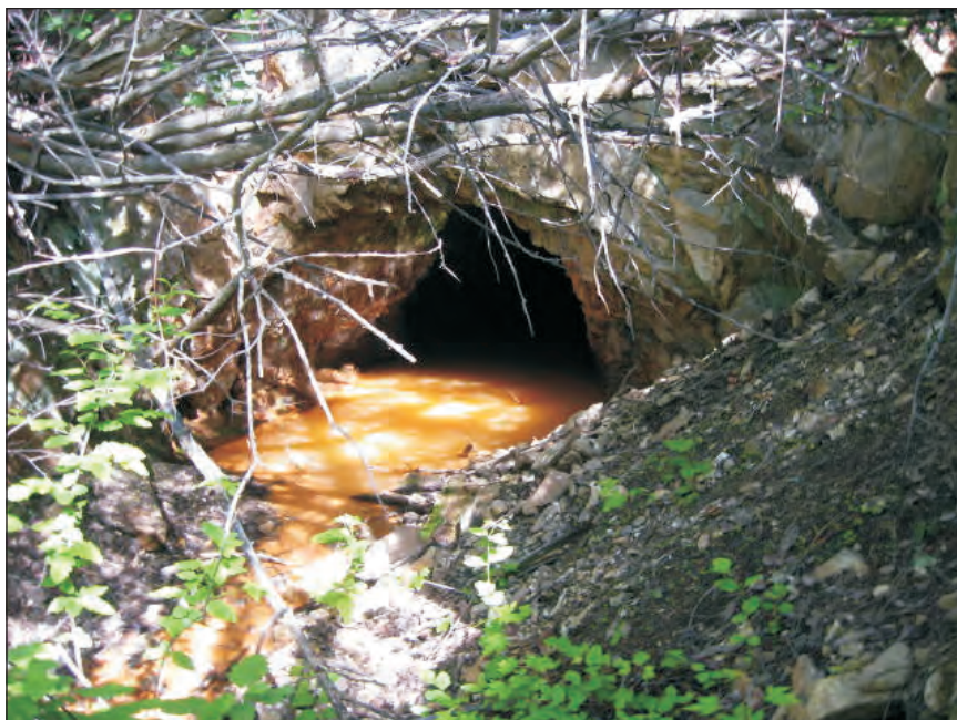
Figure 5. Acid mine drainage at the First Thought lower adit (No. 3), June 2010. Water is 4 feet deep. View is to the East.
