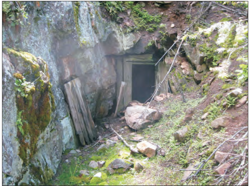
Figure 11. Portal of the upper adit of the Sonny Boy mine. The adit is open 65 feet to the heading, at which point an unmarked raise drops to the haulage level. View is to the southeast.
