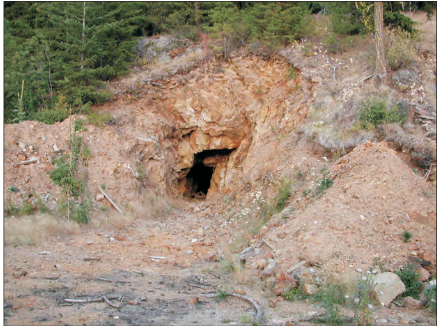
Figure 7. First Thought No. 2 level adit. The drift crosscuts the vein's hanging wall 50 feet from the portal. It is caved after that point. View is to the east.
