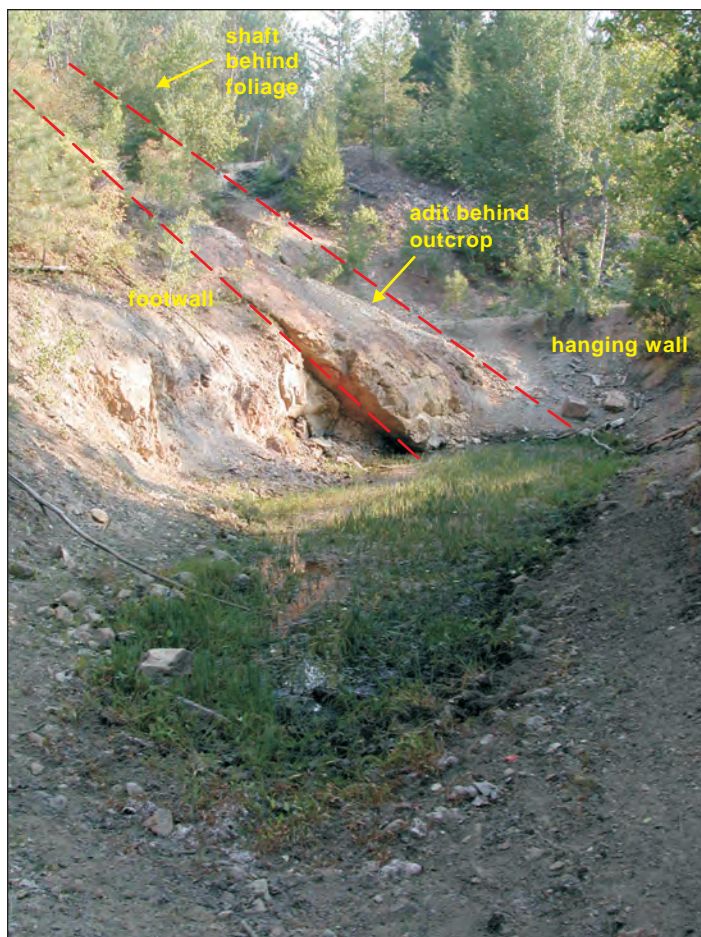
Figure 9. Circa-1980 excavation accessing the Last Chance vein outcrop dipping steeply west. Water exceeds state standards for cadmium, copper, lead, and zinc. View is to the south.
