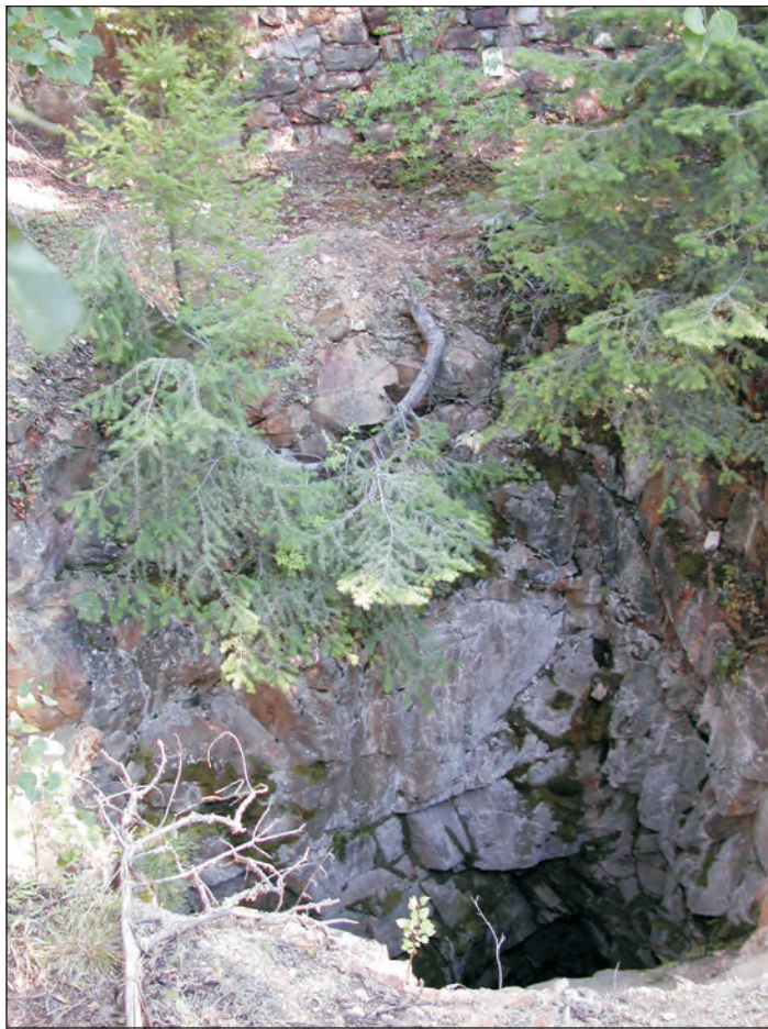
Figure 20. Site of the double compartment vertical shaft at the Fourth of July mine, caved 50 feet below the surface. View is to the east.
