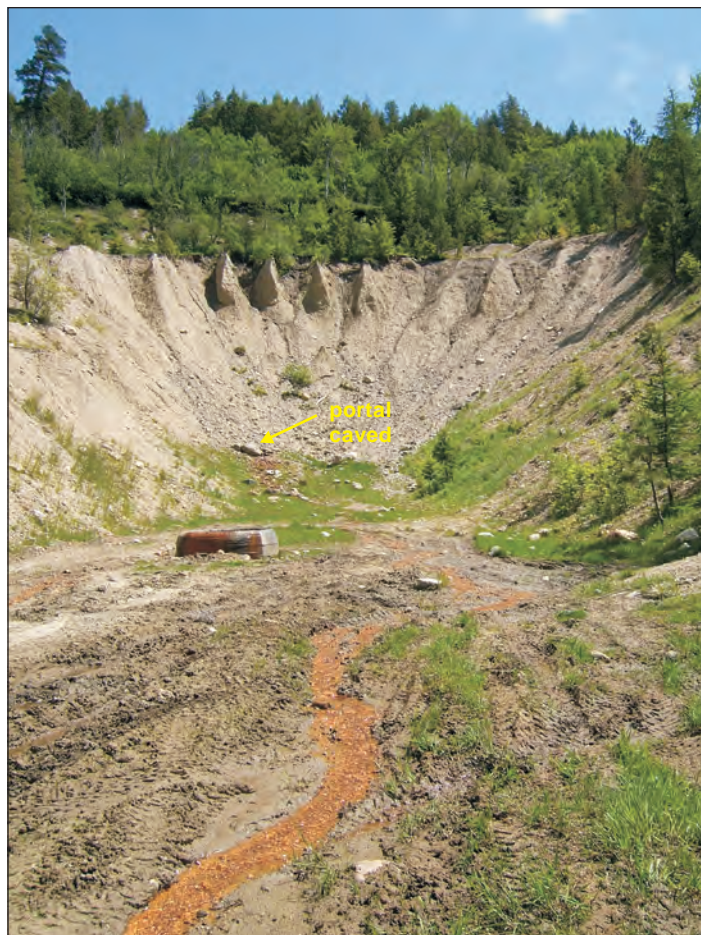
Figure 15. Overview of the Arlington site. Acid mine drainage emanates from the lower adit at the foot of the highwall. View is to the east. The mill site lies 100 feet behind the photographer's position.
