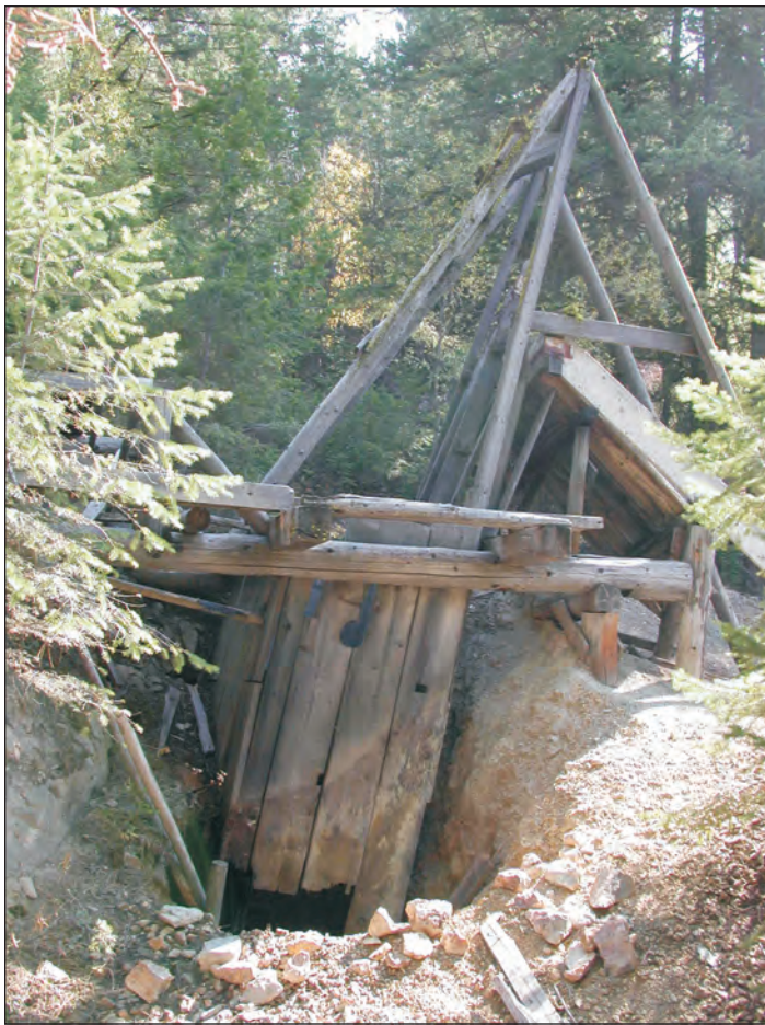
Figure 19. Inclined shaft at the Fourth of July mine, caved 10 feet below surface. Vein dips 65E.
